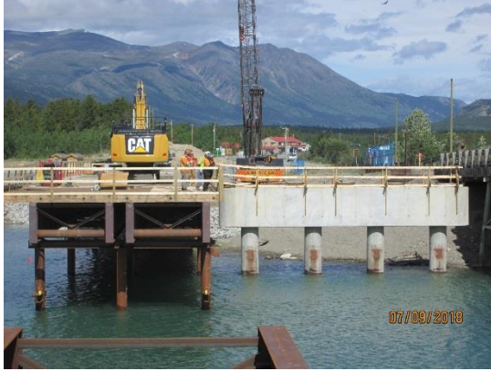
Fig. 11. Construction – Pier Cap
