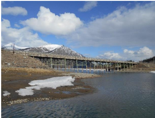
Fig. 1. Existing Bridge – Side View
