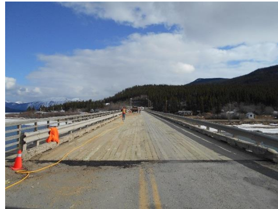
Fig. 2. Existing Bridge – Deck View
