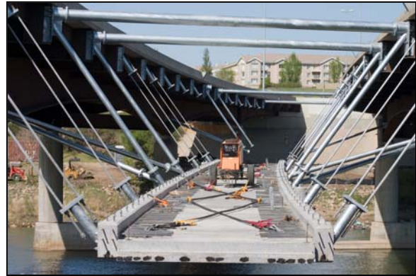
Figure 2.8 – Pedestrian Bridge Support at Pier
