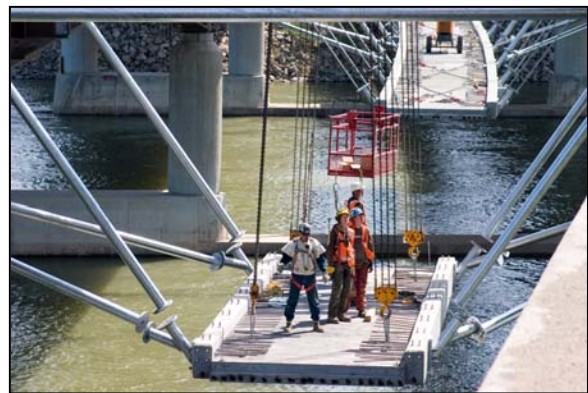
Figure 2.9 – Pedestrian Bridge Support Between Piers
