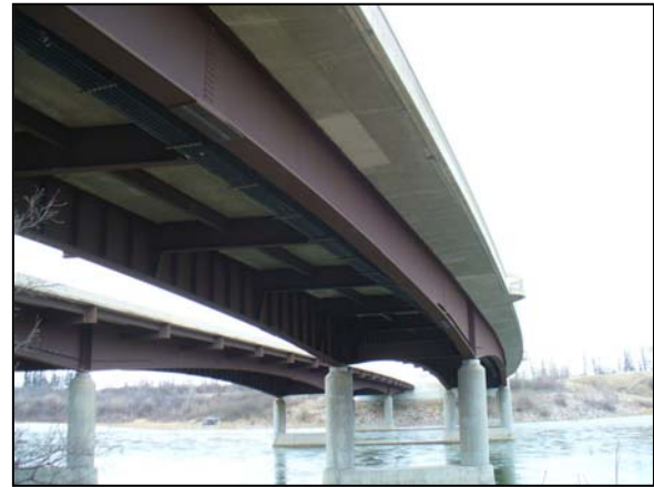
Figure 1.2 – Circle Drive Bridge
