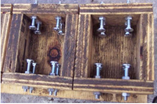
FIGURE 2: Formwork for concrete blocks with anchor bolts
