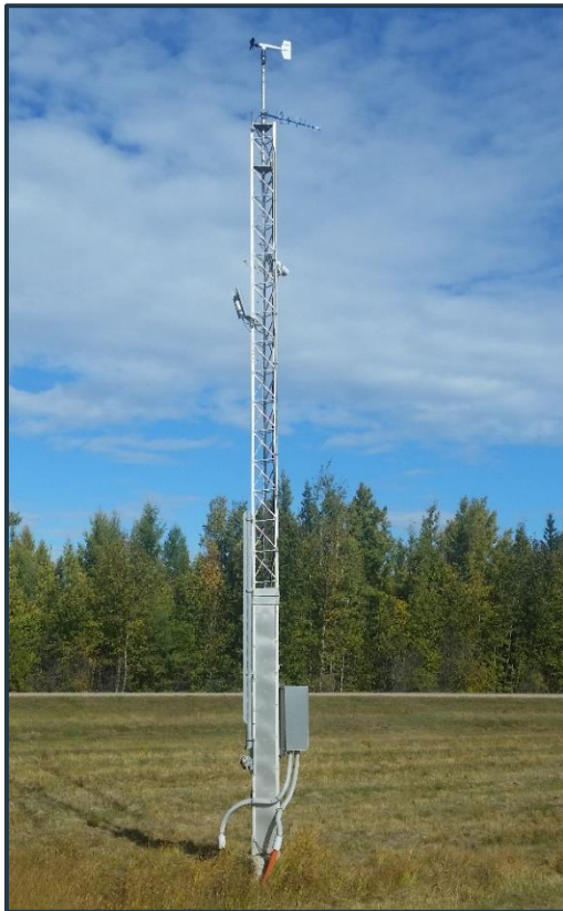
Figure 1: Road Weather Information Station (RWIS) collects atmospheric and pavement temperature data along the highway
