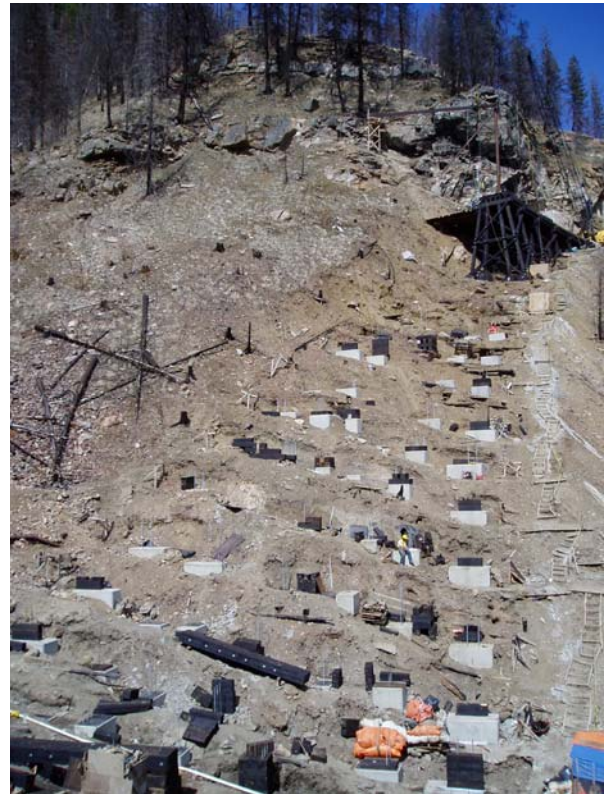
Figure 15. Highline on curved trestle 4
