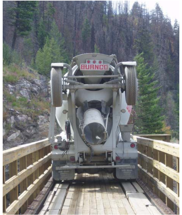
Figure 11. Concrete delivery to trestle 11
