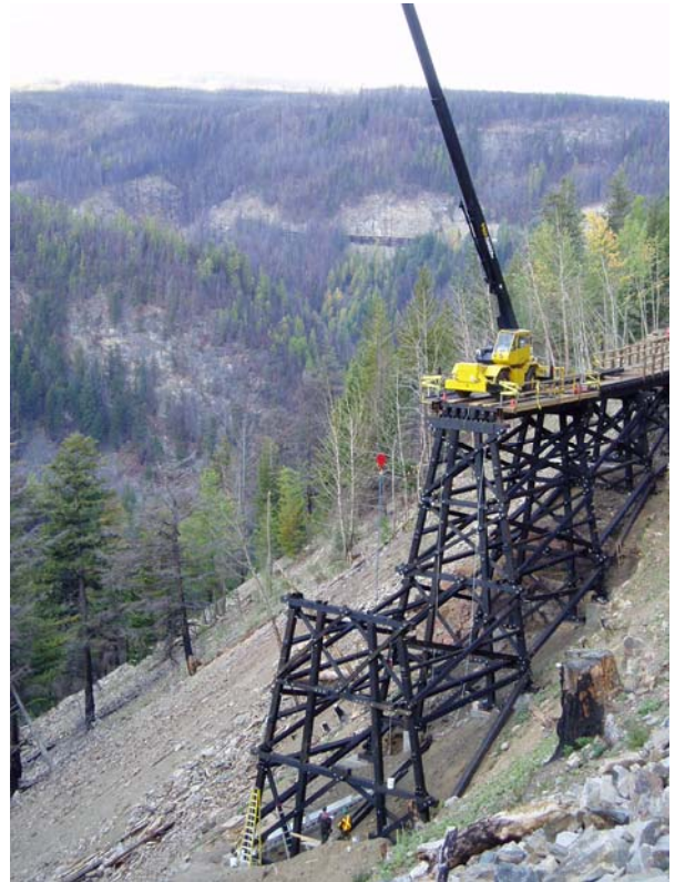
Figure 13. Rubber tired crane on trestle 11
