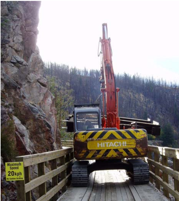
Figure 20. Delivering bent sections to trestle 15 from staging area
