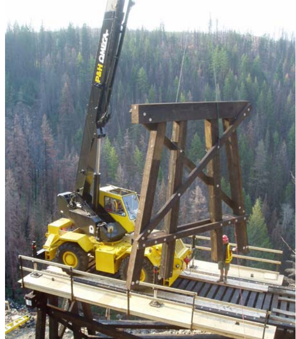
Figure 19. Placing bent sections with crane at trestle 11
