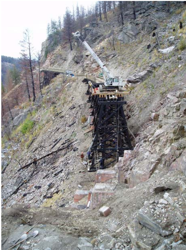
Figure 12. Tracked crane on trestle 14
