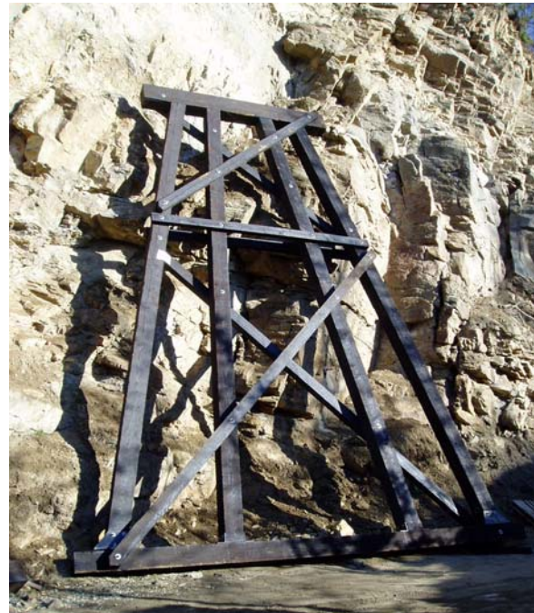
Figure 21. Prefabricated bent sections for trestle 4 in staging area
