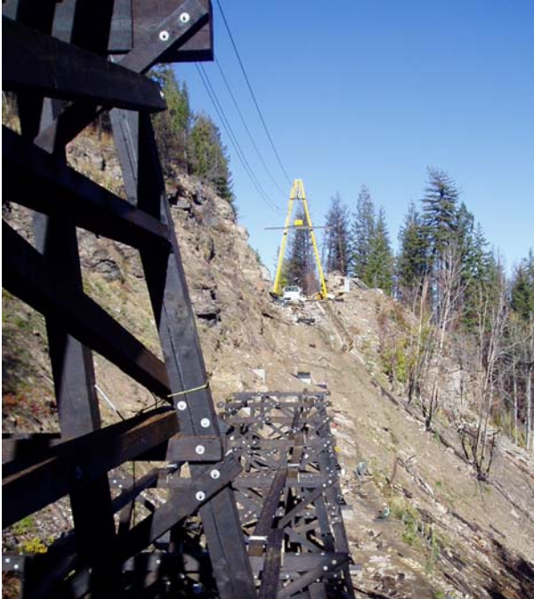
Figure 18. Assembling bent with highline at trestle 2
