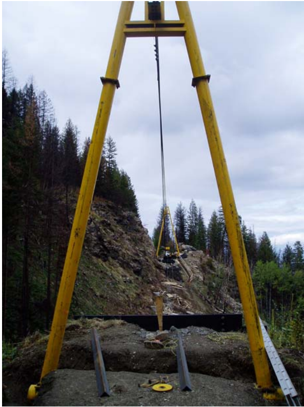
Figure 14. Highline on tangent trestle 2
