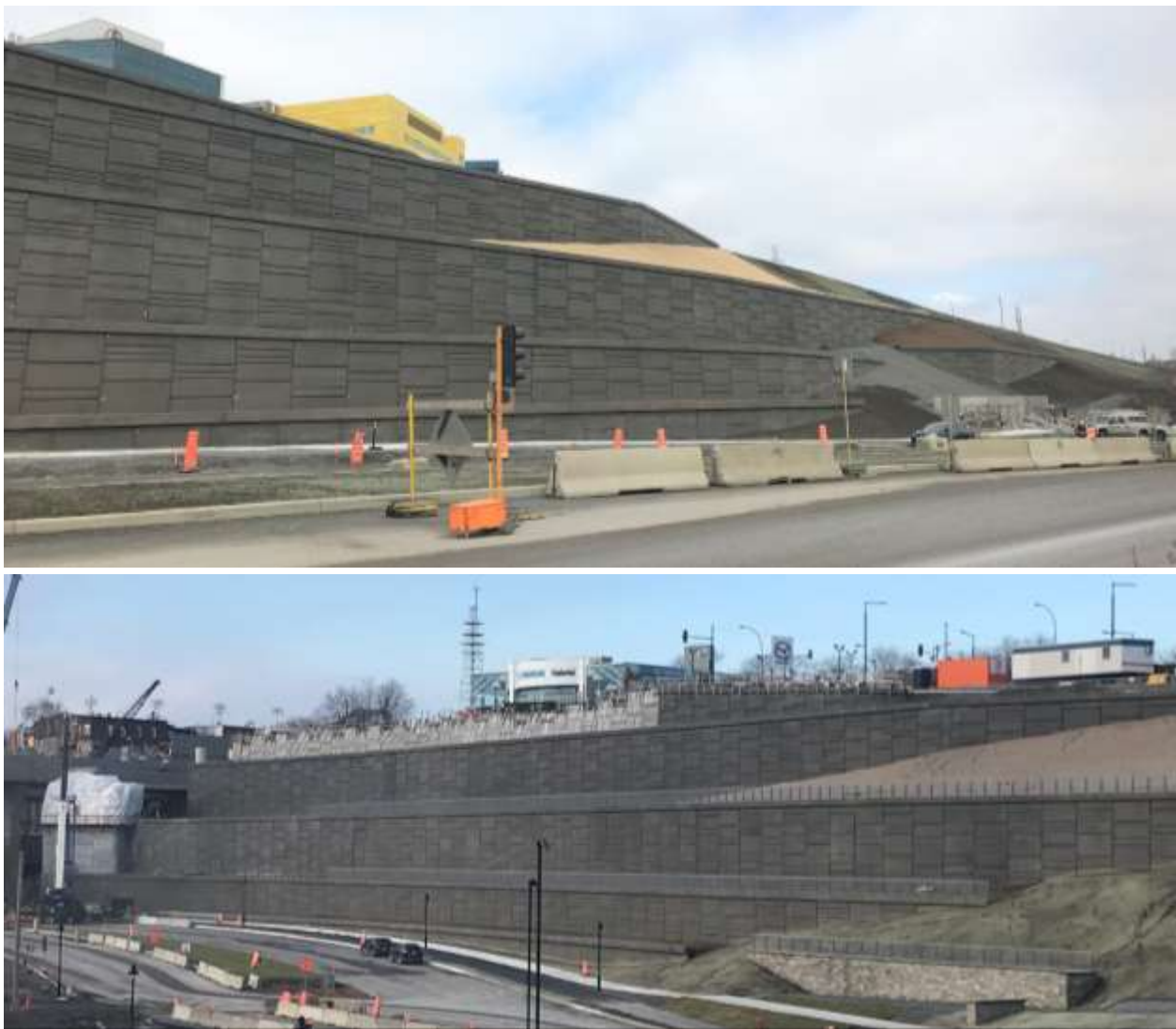
Fig-14. Photos of Completed Wall
