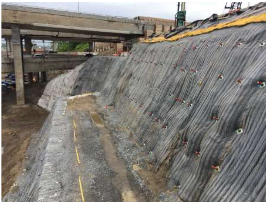
Fig- 8. Completed Soil Nail Stabilized Excavation Slope
