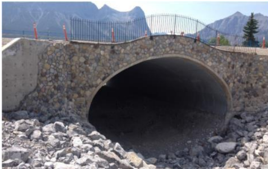
Figure 19 - Cougar Creek Crossing with Rehabilitated Soil
