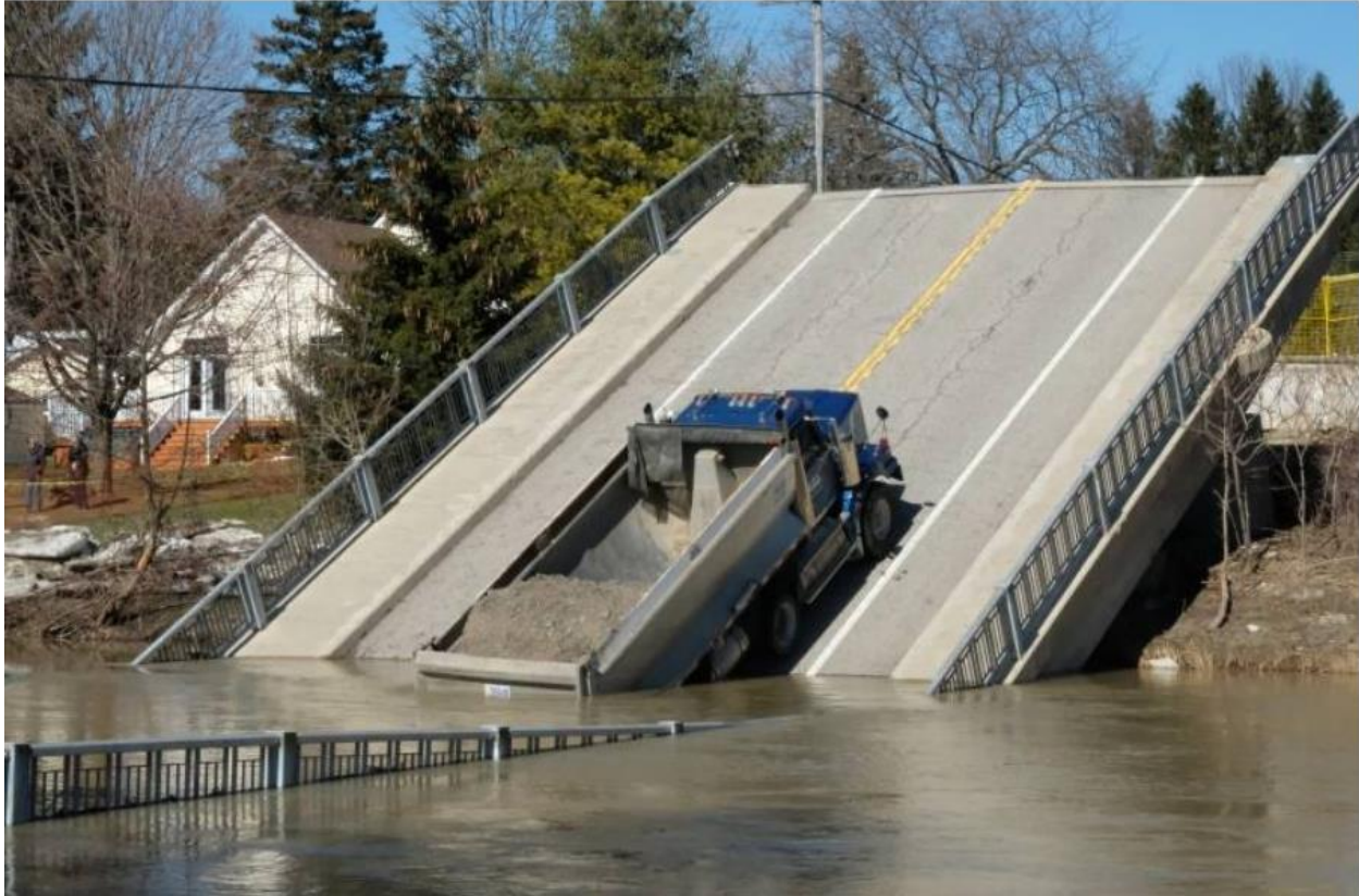
Figure 1 - Bridge Failure During an Extreme Hydraulic Event (Duhatschek, 2018)
