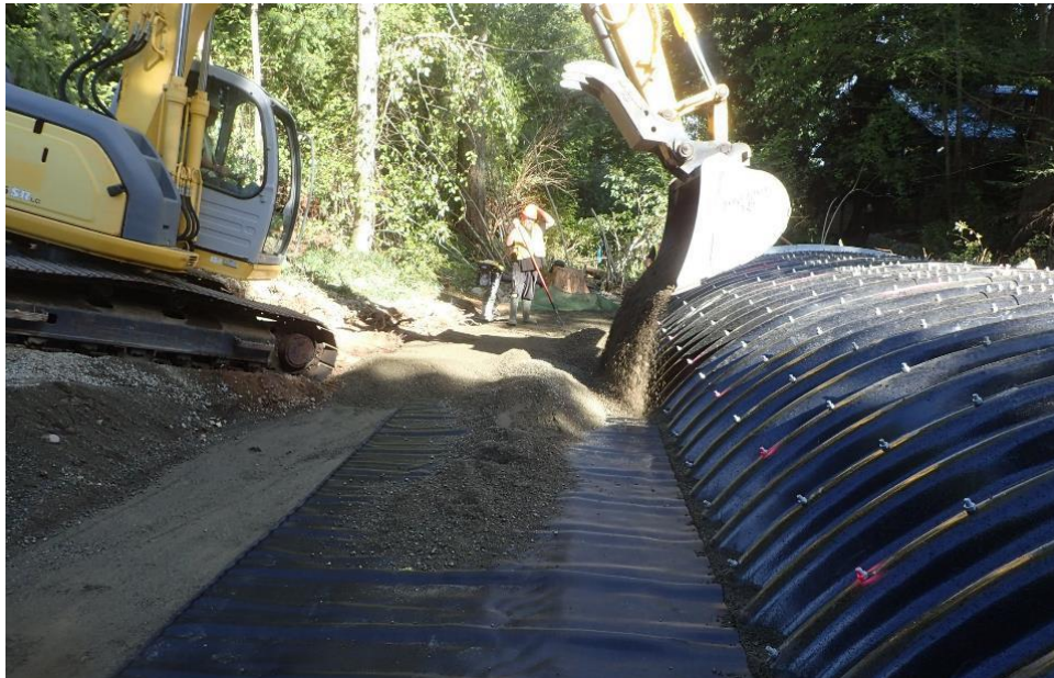
Figure 8 - GRS being Backfilled (Wong, 2016)
