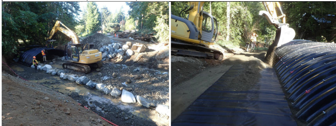
Figure 11: GRS Buried Structure During Construction (photo courtesy of Sean Wong, BCMOTI)
