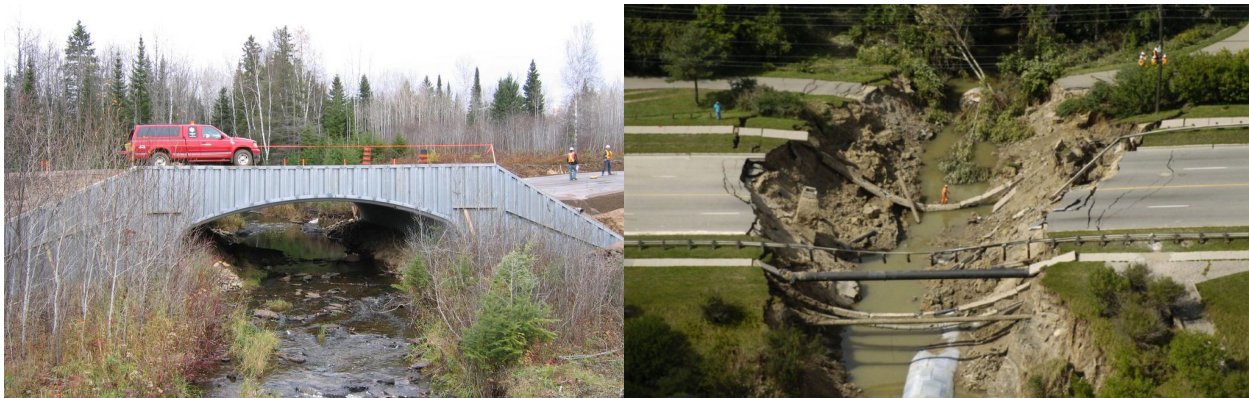
Figure 8: Adding Resilience to Avoid Backfill Washout
