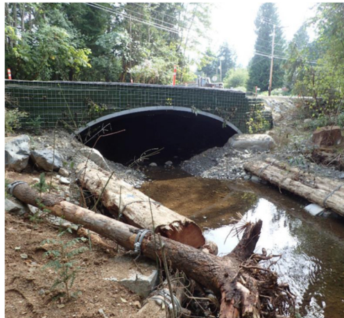
Figure 12: Constructed GRS Buried Structure (photo courtesy of Sean Wong, BCMOTI)
