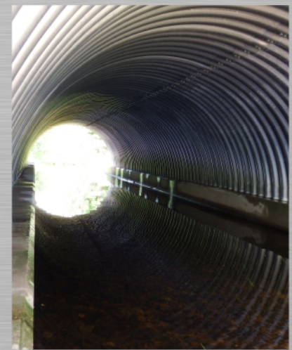
Typical aluminum structural plate bottomless arch on concrete footings.
