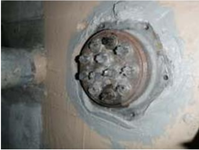
Figure 21. Post-Tension Impregnation Material leaking from the far end of 2 strands of a tendon (255 ft from point of impregnation)
