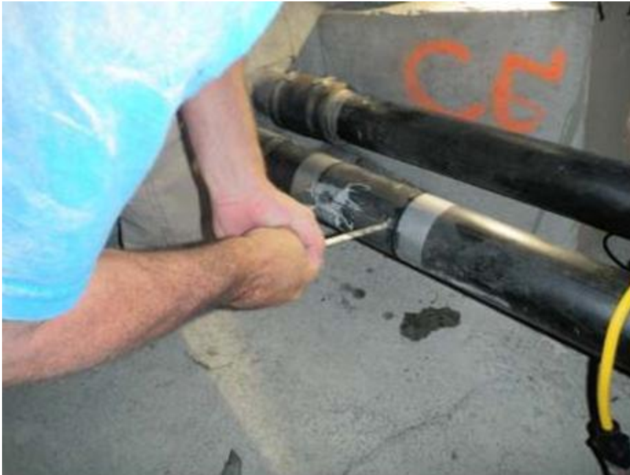
Figure 23. Removal of plastic duct after cutting
