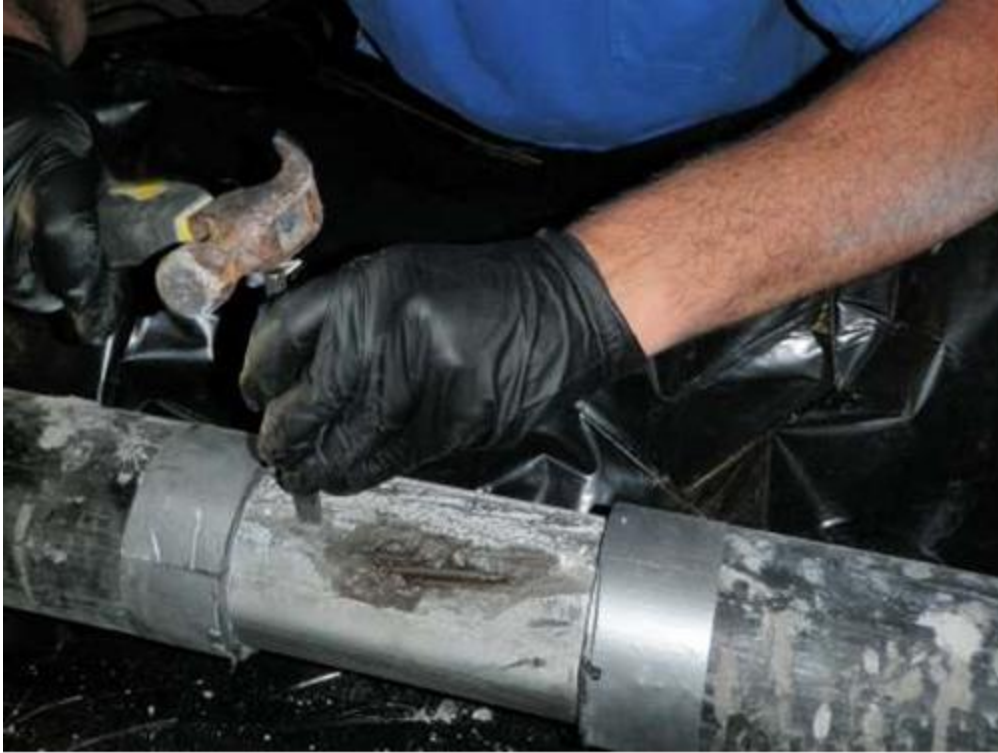
Figure 24. Chipping grout to expose strands and observe the level of saturation
