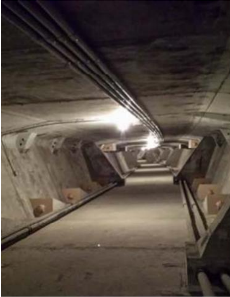
Figure 18. Interior view of FDOT bridge showing post-tensioned cables and anchorages
