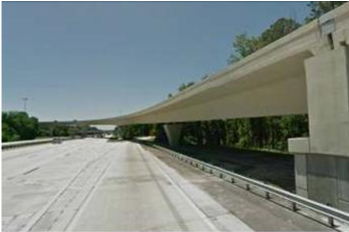
Figure 17. Street view of FDOT bridge
