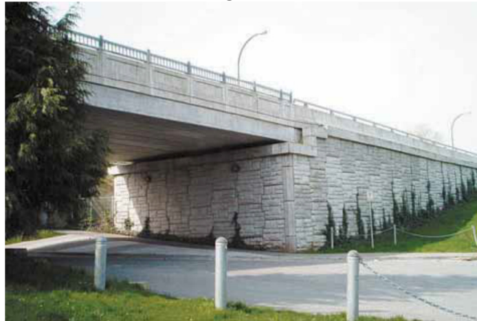
Windemere Overpass. Vancouver, BC
