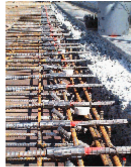
Galvashield ® XP anodes installed along joint interface
