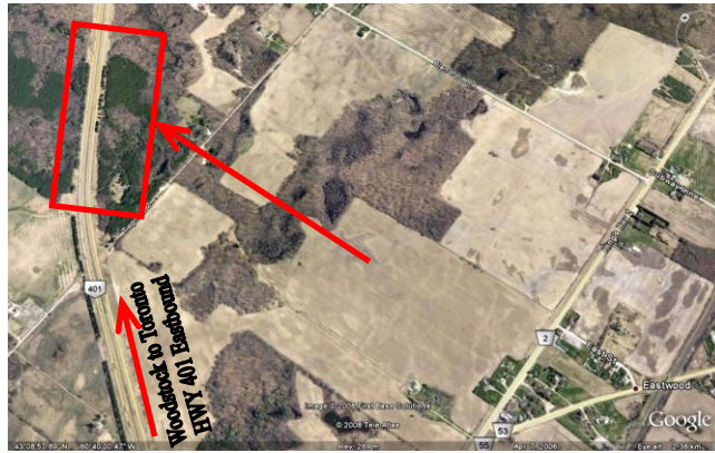
Figure 6- The CPATT site on HWY 401, between the exits 238 and 250 on Eastbound
