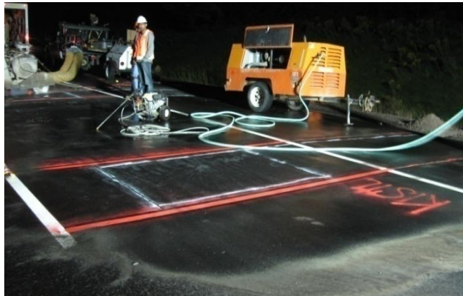
Figure 7- Installation of the WIM sensors
