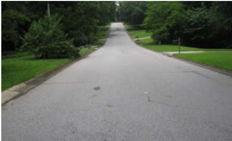
Figure 2. Example of appearance of a weathered asphalt pavement with SRI about 6.
