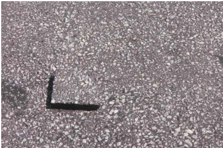
Figure 3. Example of LCAP pavement of ongoing research.
