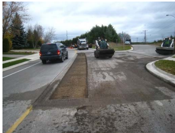
Figure 10. Repairs of new binder course that incorporated high amount of RAS.
