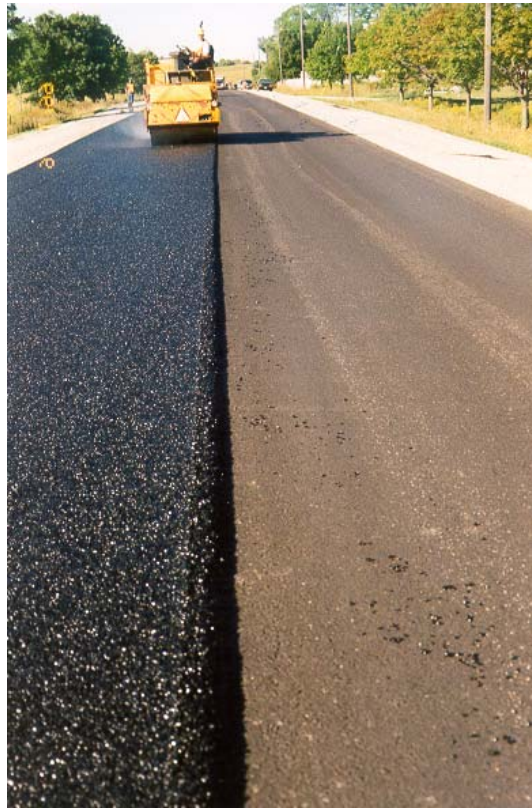
Figure 7 – SMA paving on Simcoe Road in the Region of Durham, Ontario in 1999.
