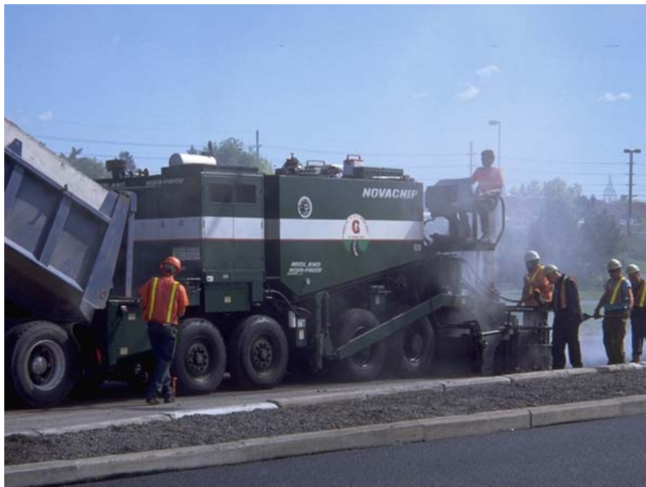
Figure 6 – Application of Nova Chip on Anderson Street, Whitby in 1998
