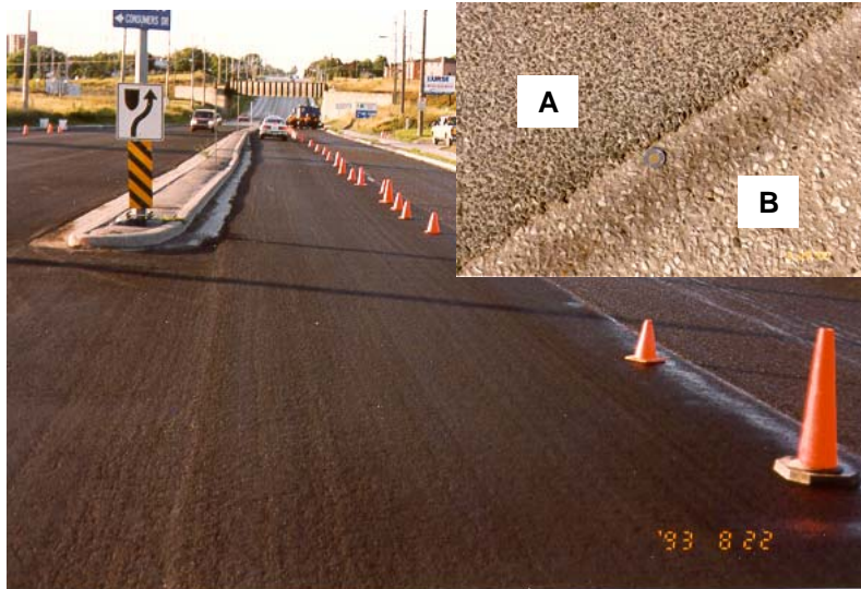
Figure 4 – Application of microsurfacing on Thickson Road in Whitby, Ontario in 1993. The close up compares the microsurfacing surface texture with (A) the existing polished HMA surface texture (B).
