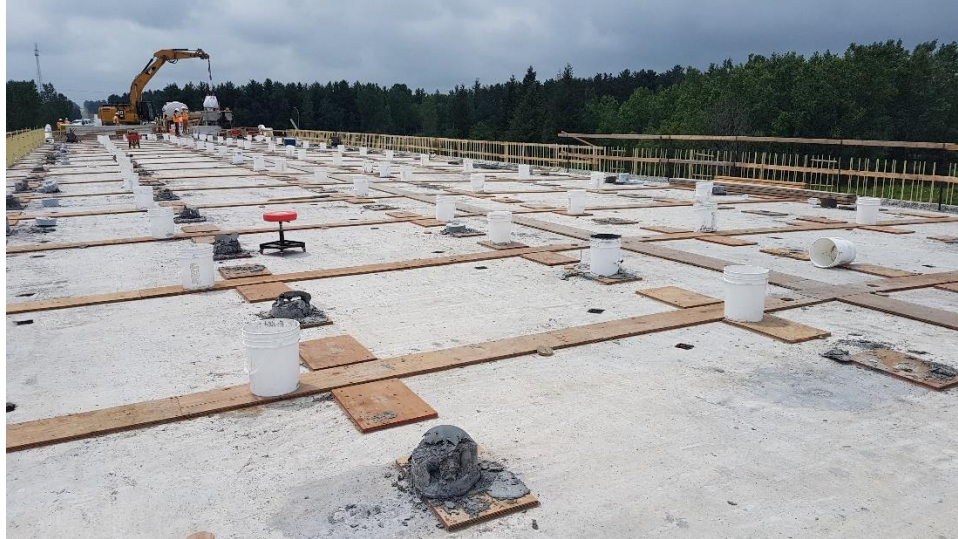
Figure 4: Typical Field-cast Joint Placement
