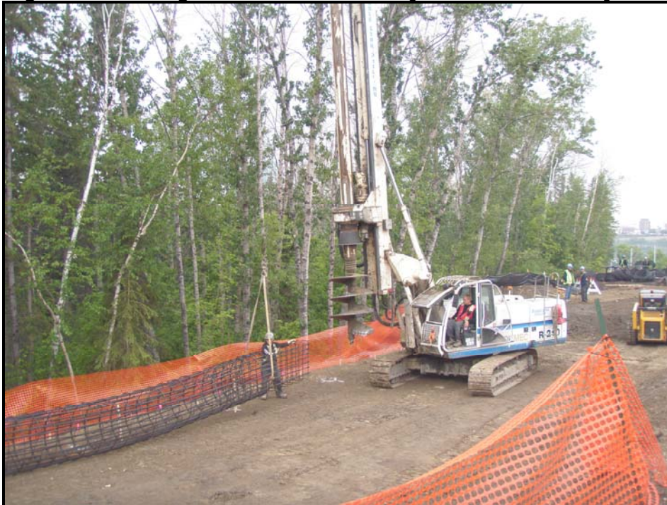
Figure 4: Retaining Wall 2 Construction Adjacent to River Valley
