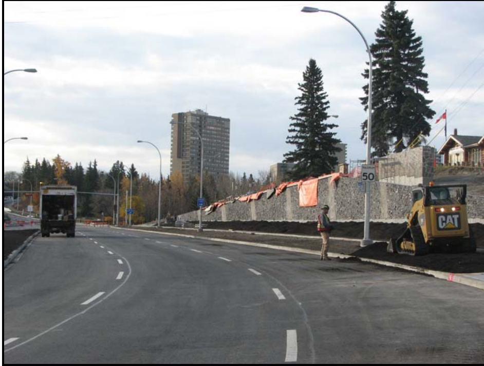
Figure 3: Retaining Wall 1 and Guy Wire Structure
