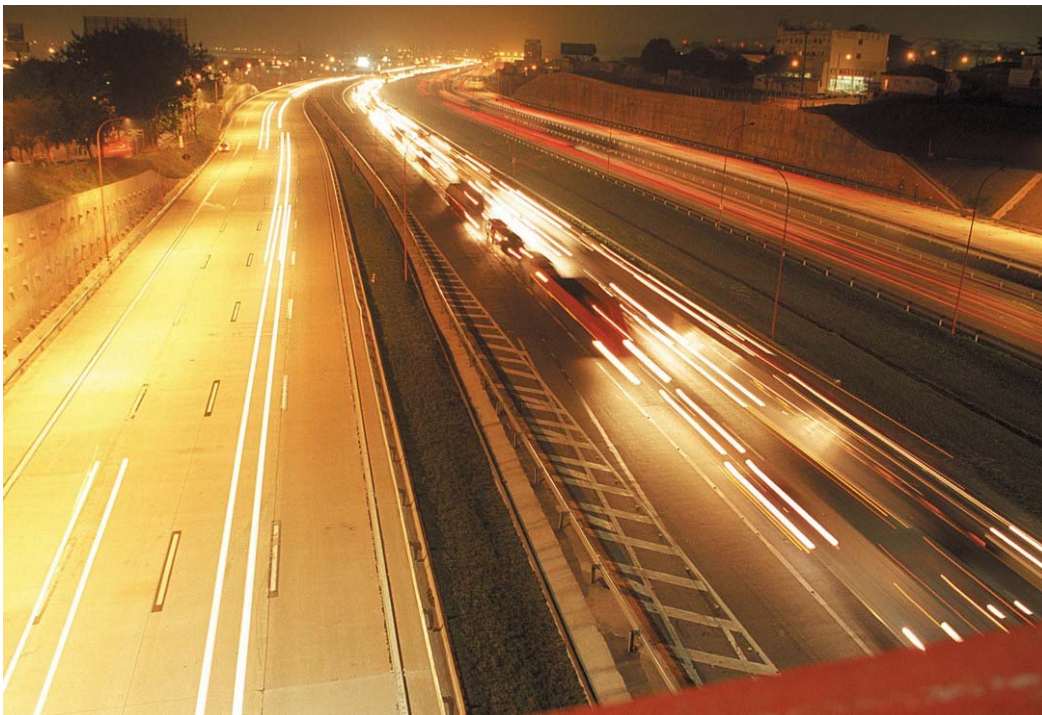
Figure 3: Night Time Picture of PCCP and ACP on Highway Castello Branco - São Paulo State, Brazil
