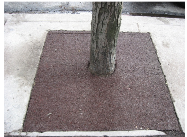
Image 6: Pedestrian Safety – tree pits – potential trip hazards, and using flat tree pits that provide mulch for trees
