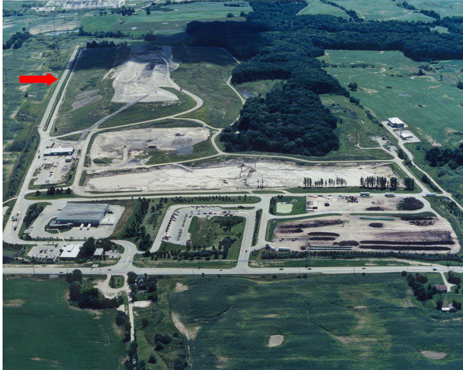
Figure 1: Regional Municipality of Waterloo’s waste management facility
