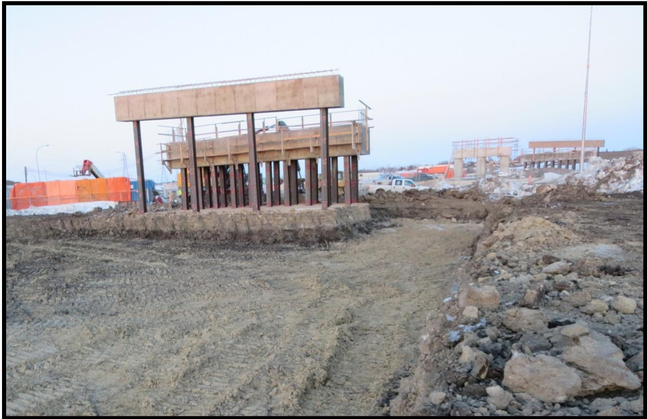
FIGURE 8: COMPLETED SUBSTRUCTURE UNITS
