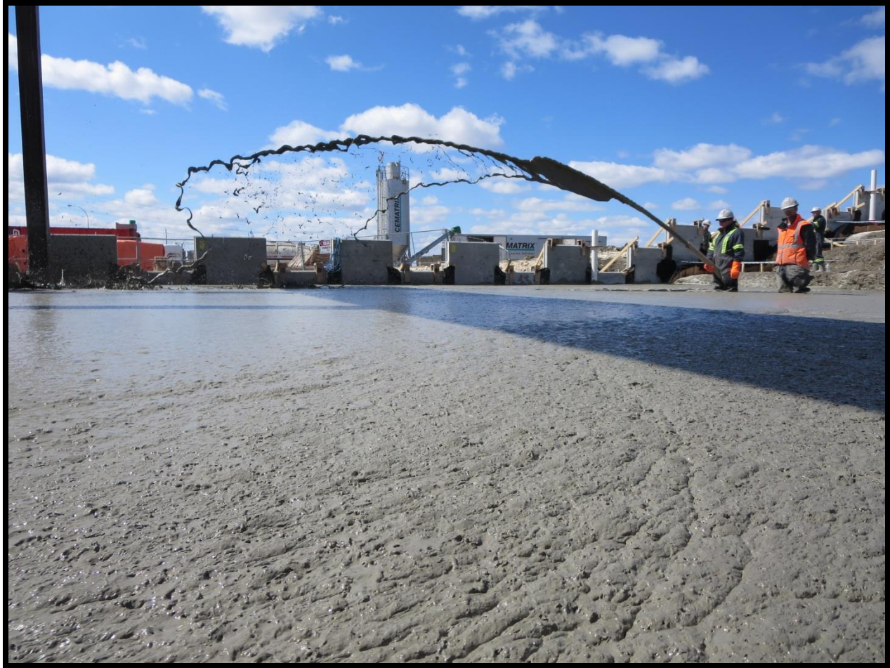
FIGURE 15: POURING LIGHTWEIGHT CONCRETE BACKFILL
