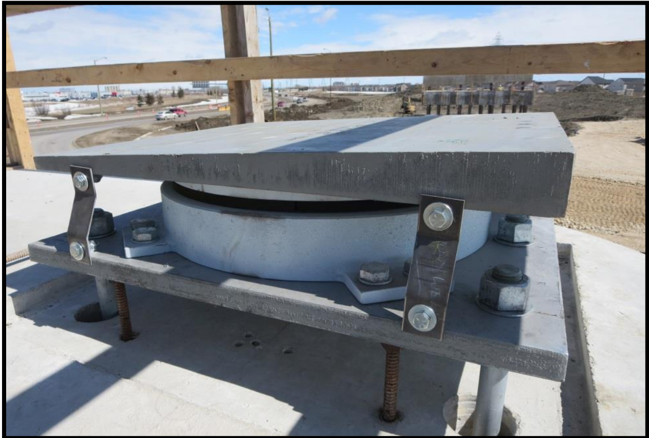
FIGURE 12: POT BEARINGS PRIOR TO GIRDER ERECTION AND FINAL GROUTING
