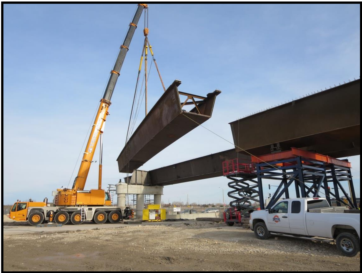
FIGURE 11: GIRDER ERECTION
