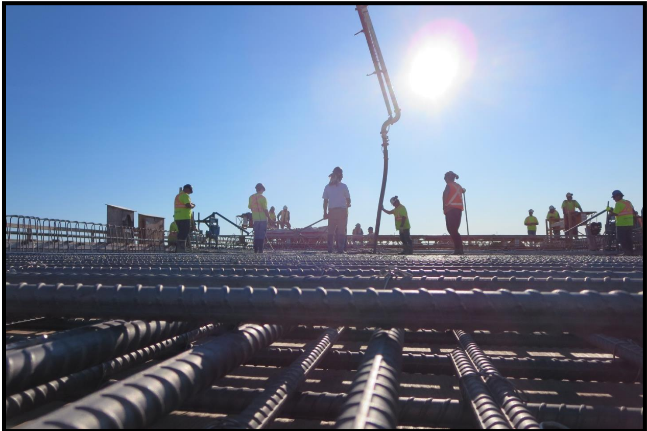
FIGURE 13: DECK CONCRETE PLACEMENT
