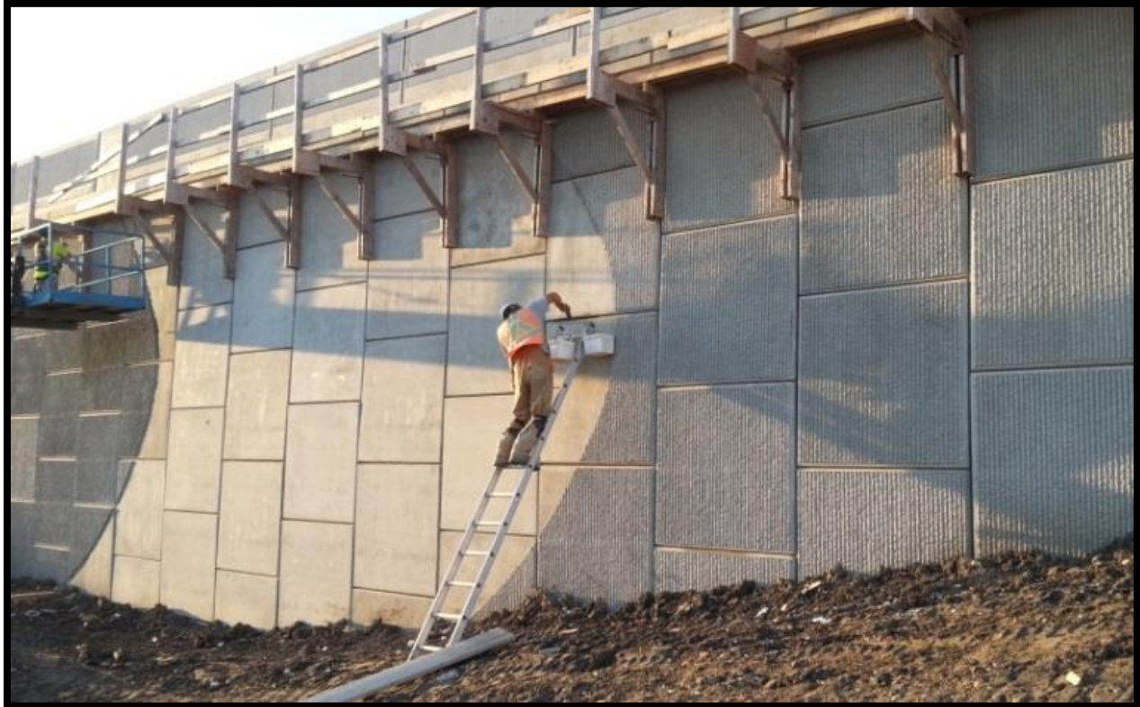
FIGURE 14: MSE WALL SHOWING AESTHETIC TREATMENT
