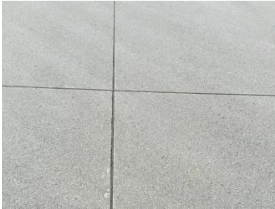
Photograph 3 – Properly sawcut and sealed longitudinal and transverse joints.
