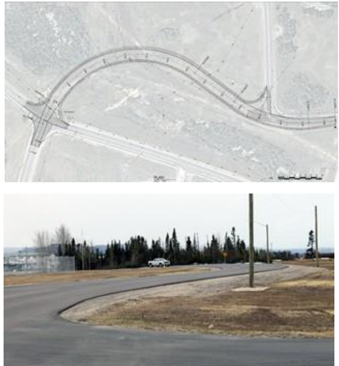
Figure 8 CFB Goose Bay, Vulcan Road Extension
