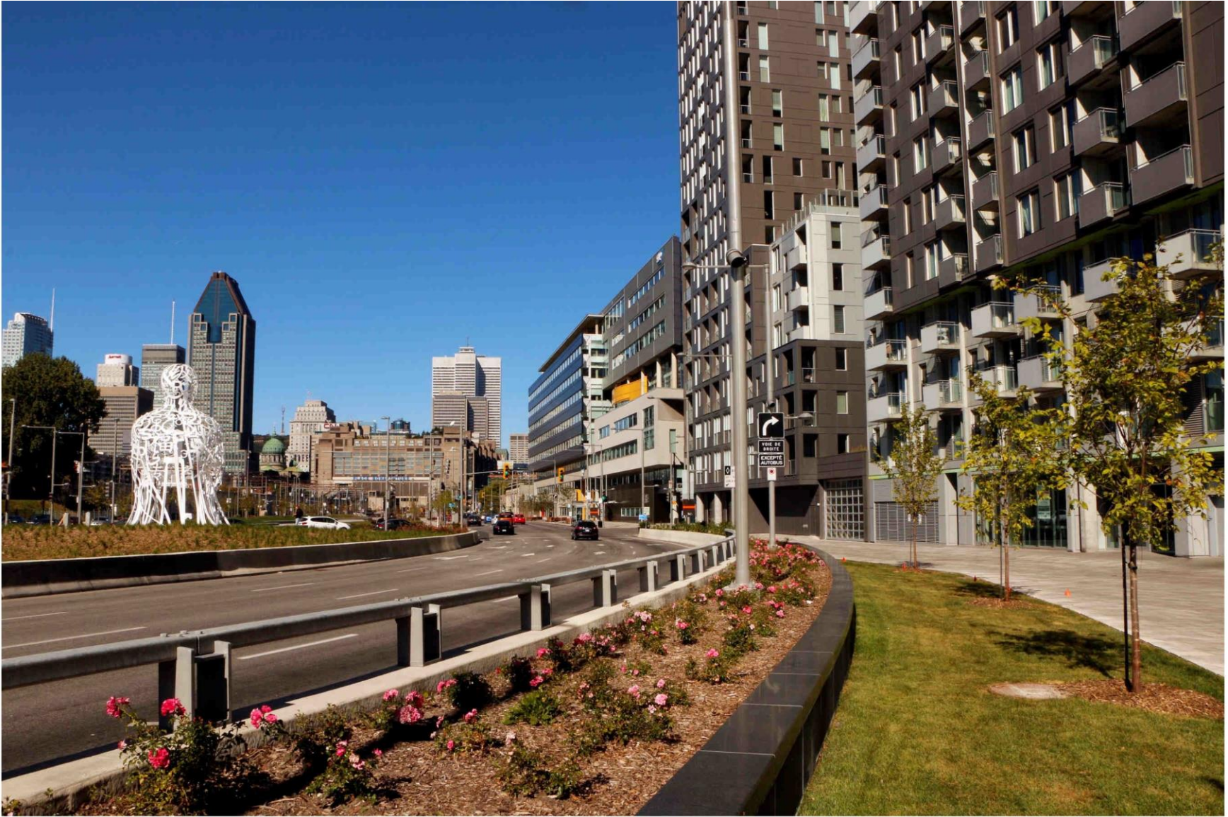
Bonaventure 2B: View from the Duke Ramp, looking north, 2017
