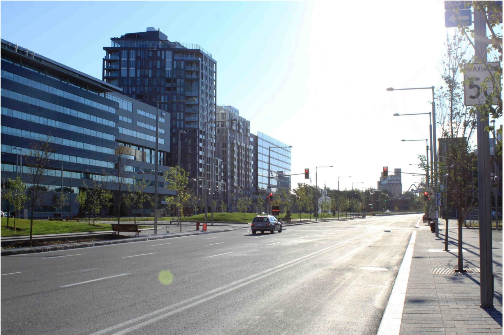
Bonaventure 1B: View along Nazareth Street, looking south, 2017
