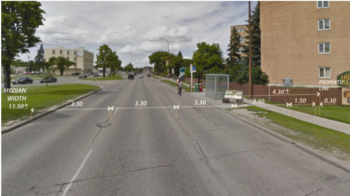
Figure 1 – Previous conditions along Pembina Highway
