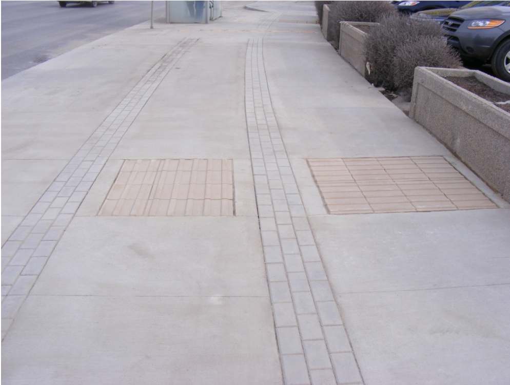
Figure 5 – Cycle Slab pavers and paving bands
