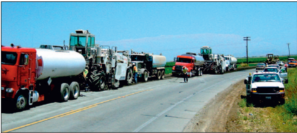
Figure 1.1-1 typical Cold In-place Recycling project
