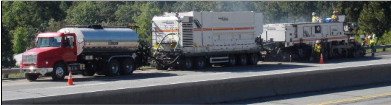
Figure 3.1-1 Bitumen truck, slurry mixer and recycler
