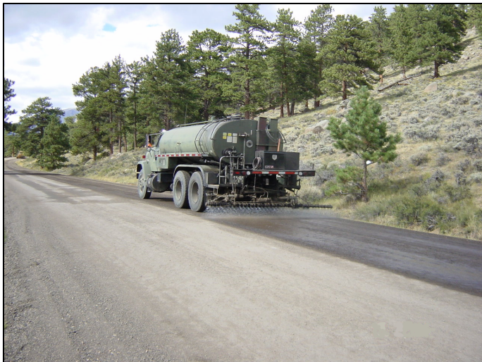
Figure 3.4-1 fog sealing operation
