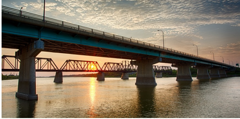
Figure 8 – Diefenbaker Bridge Rehabilitation
