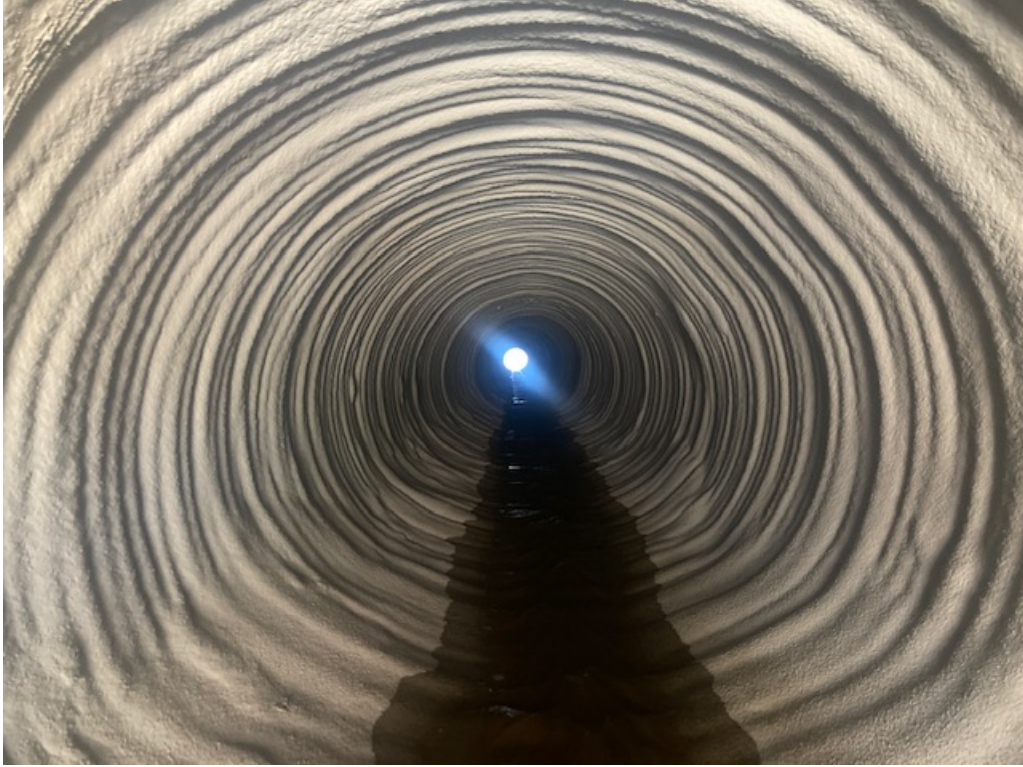
Figure VIII – Photo of Site ND07 After Final Application
