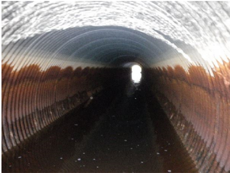
Figure I: Culvert Rehab Candidate, fully backwatered
