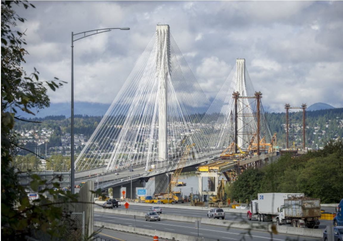
The Port Mann Bridge, as seen from north Surrey.
