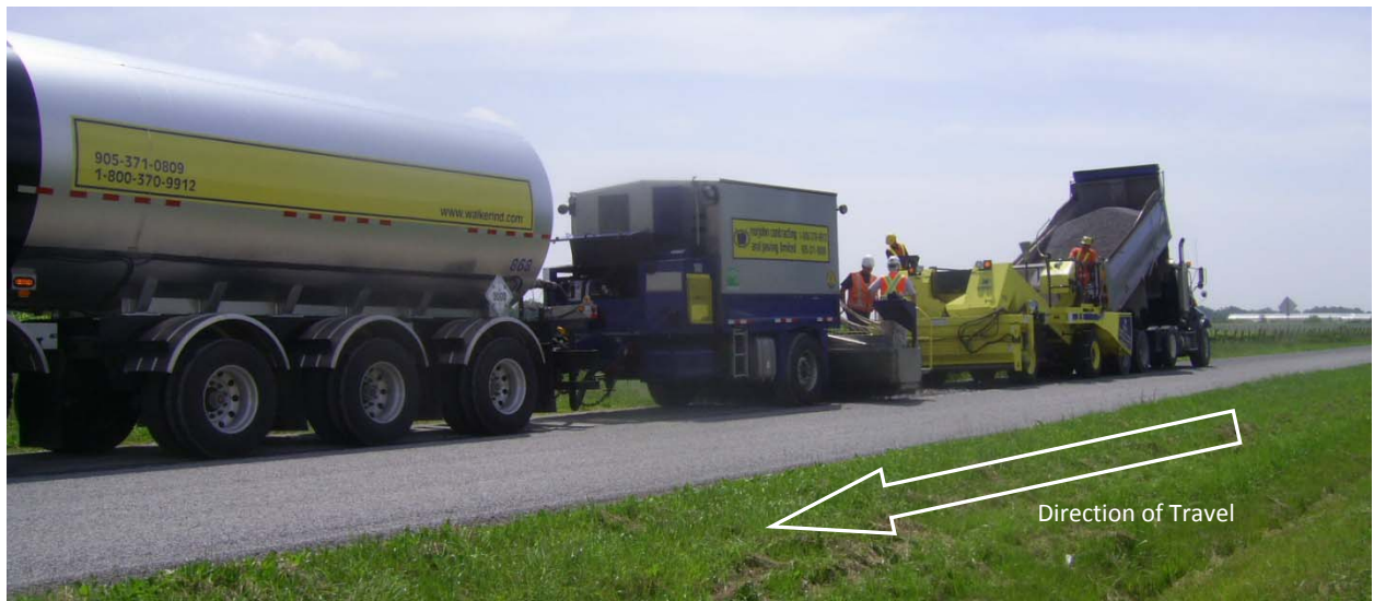
Figure 7. Tanker, FiberMat™ machine, chip spreader and aggregate delivery truck
