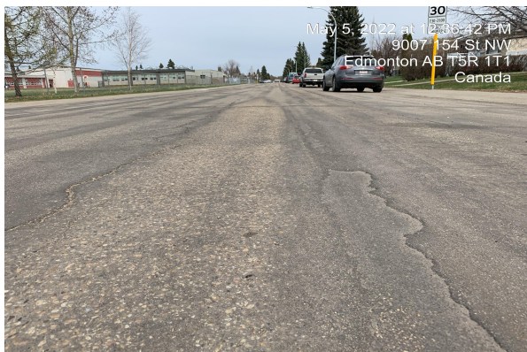
Photos 5 to 8 show the condition of MSF after 6 years. Some ravelled areas between the wheelpaths were observed.
