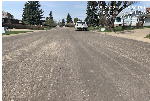
Photo 17 : Pre-treatment condition (left). Photo 18: MSF condition after the first year. A drag mark was visible in most locations (right)
