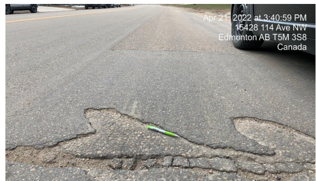
Photos 13 and 14: Two localized failed MSF locations
