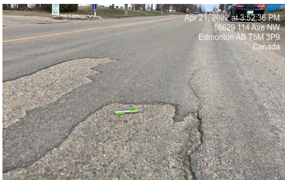
Photos 13 and 14: Two localized failed MSF locations
