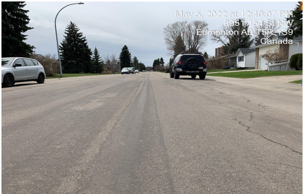
Photos 5 to 8 show the condition of MSF after 6 years. Some ravelled areas between the wheelpaths were observed.
