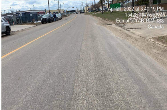
Photos 15 and 16: Area with reasonable MSF performance. Difference of surface colors between two lanes was noticed
