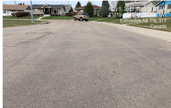
Photo 1: Ravelled areas after 8 years (left) and Photo 2: A better MSF performance in a roundabout boulevard was still effective after 8 years
