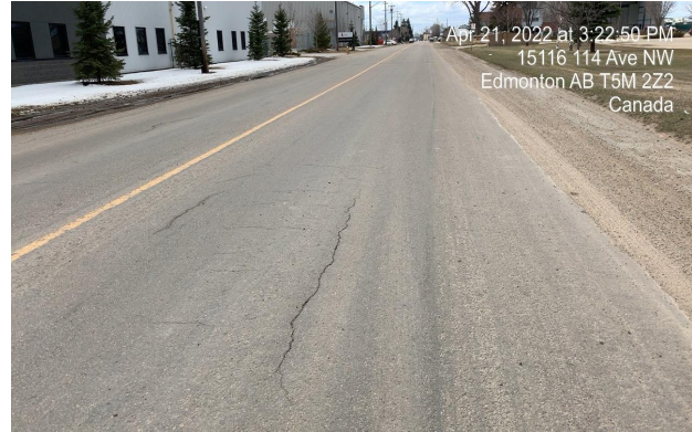
Photos 15 and 16: Area with reasonable MSF performance. Difference of surface colors between two lanes was noticed
