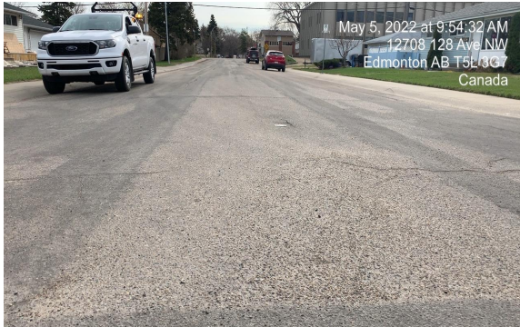
Photo 1: Ravelled areas after 8 years (left) and Photo 2: A better MSF performance in a roundabout boulevard was still effective after 8 years
