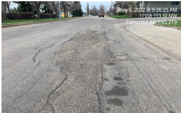
Photos 3 and 4: Delaminated MSF area (left) and difference between untreated and MSF treated surface after 7 years (right)
