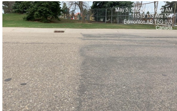
Photos 3 and 4: Delaminated MSF area (left) and difference between untreated and MSF treated surface after 7 years (right)
