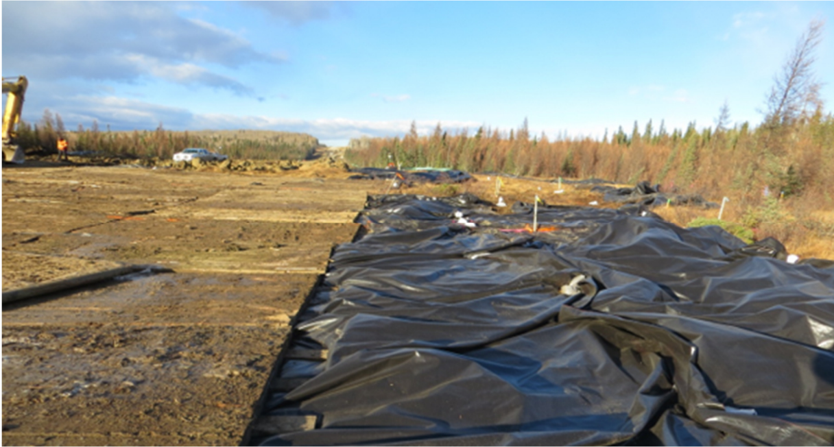
Photo 5.7: additional layers of geogrid used within subgrade layer above failure area
