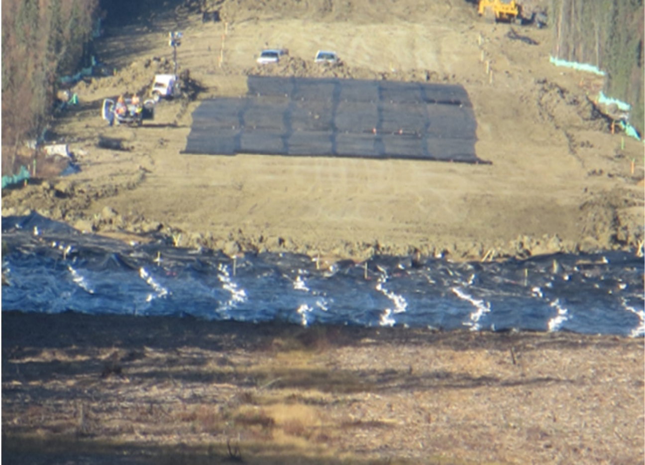
Photo 4.1: Muskeg area with geotextile and geogrid placement separated by fill material
