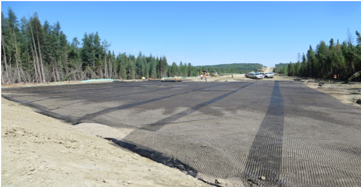
Photo 5.9: showing the fourth level of geogrid placement above the failure area
