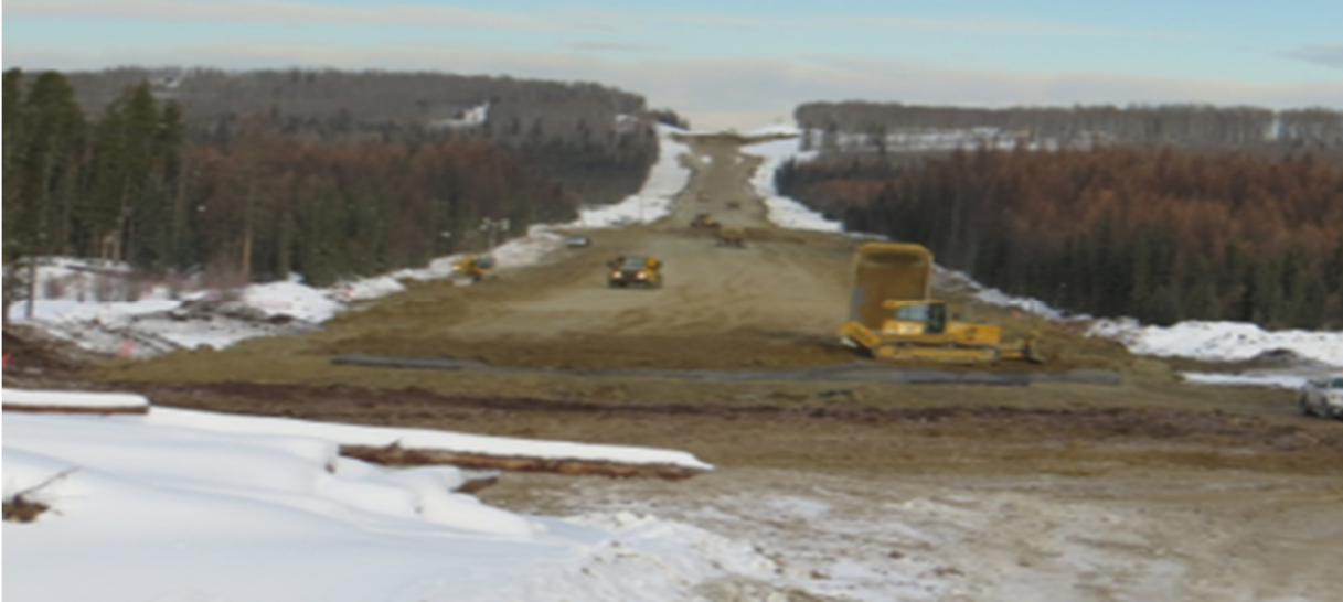
Photo 5.4: showing upper-level grade construction over geotextile and geogrid layers
