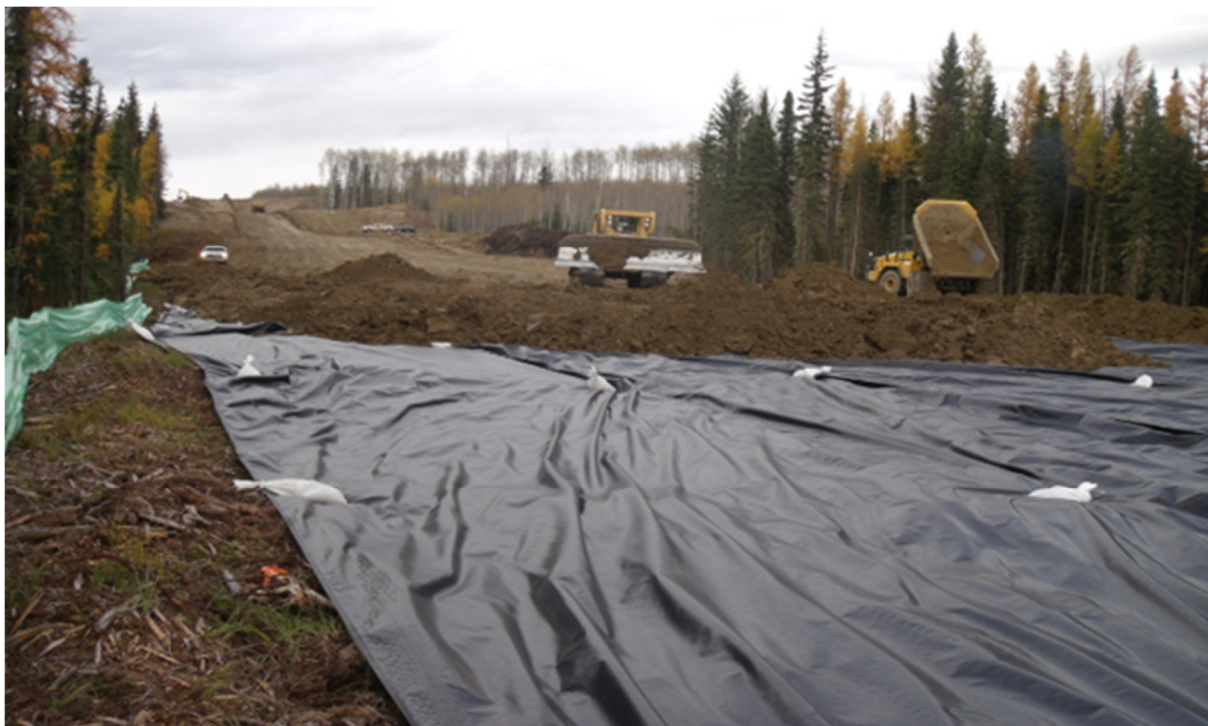
Photo 5.2: showing geotextile fabric placement and initial layers of embankment
