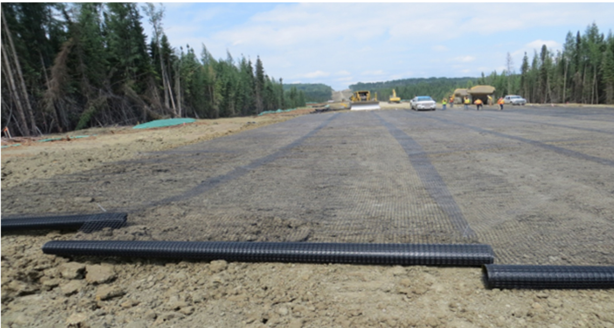
Photo 5.7: additional layers of geogrid used within subgrade layer above failure area
