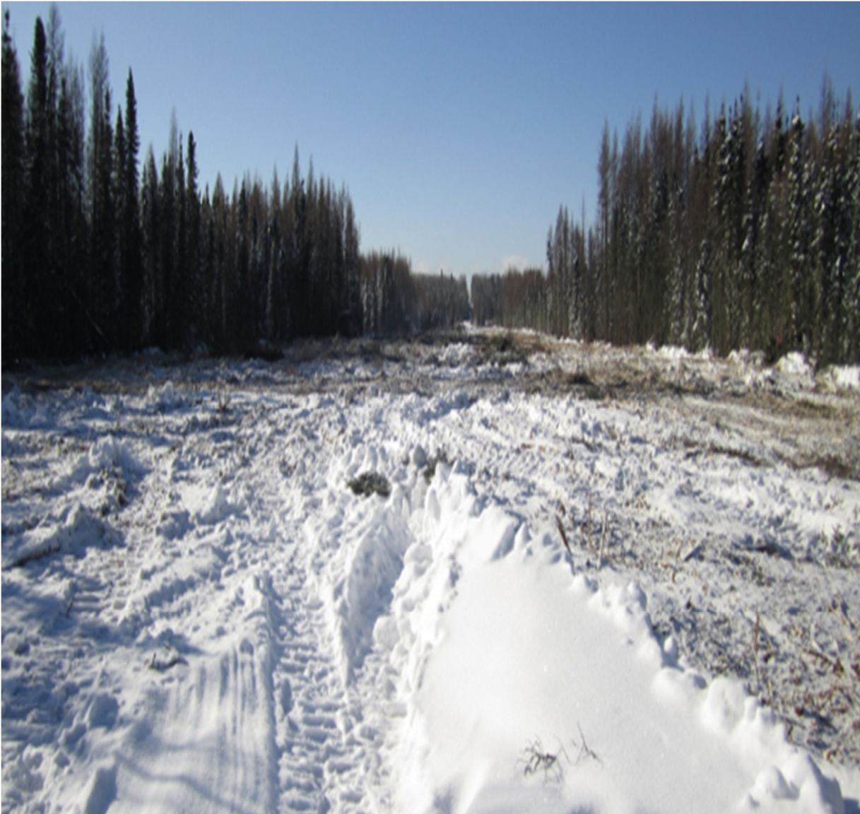
Photo 5.1: showing tree and bush clearing over muskeg areas
