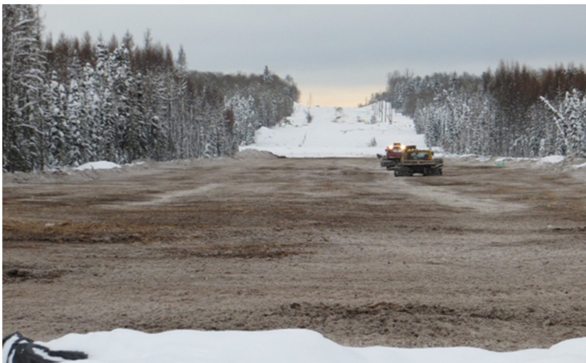
Photo 5.3: showing machine tracking to force frost deeper into the muskeg
