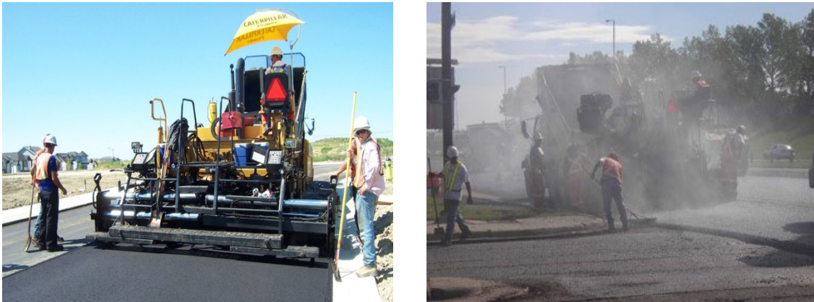
Figure 5. WMA paving (left); HMA paving (right)
