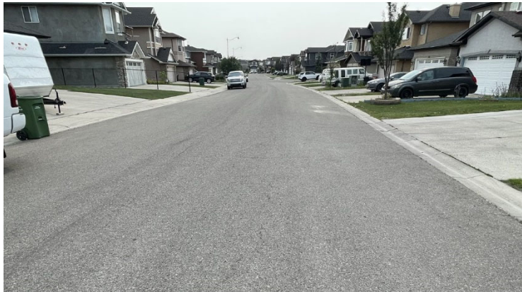
Figure 3. Typical View WARM-Foam Residential Roadway Section in 2021
