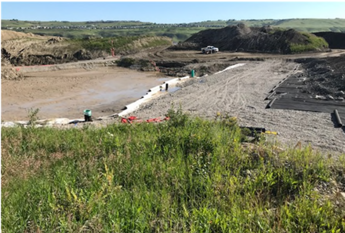
Figure 3: Drainage Blanket Construction on the South Pond
