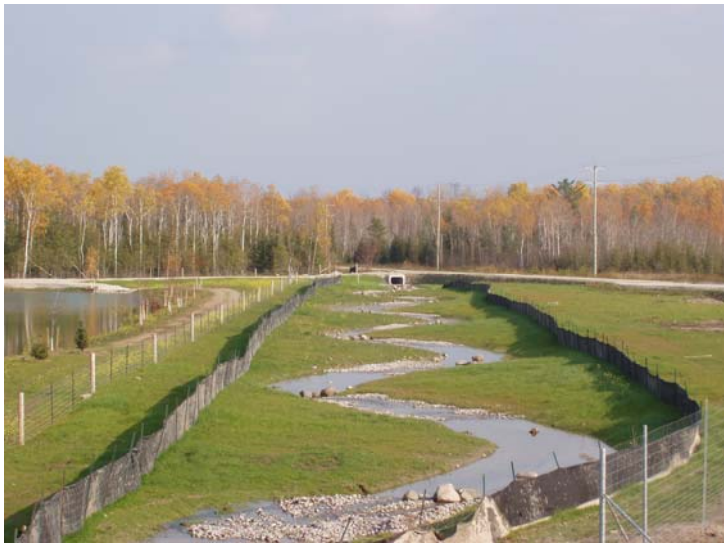
Figure 10 One of the Eight Stormwater Management Ponds:
