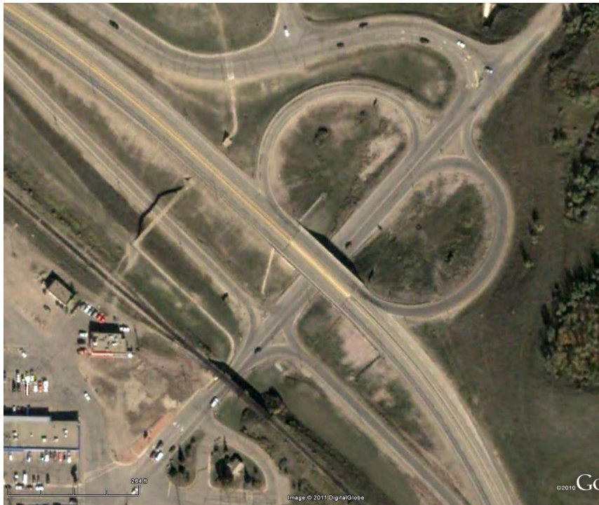
Figure 13: Google Earth Image highlighting Highway 2 and Pats Creek Road.
