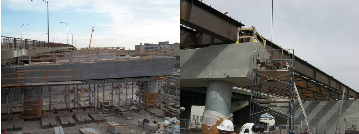
Figure 6 – Post-Tensioned Pier Cap
