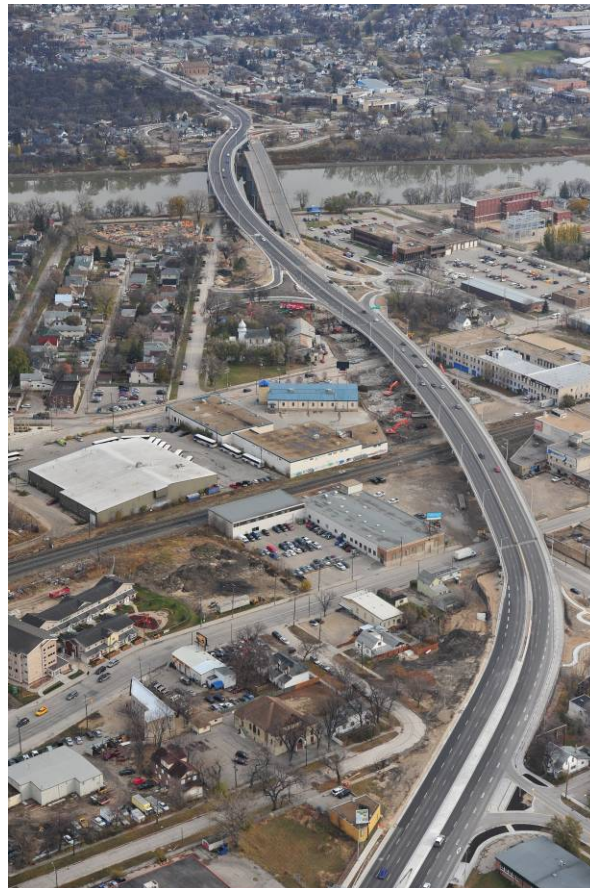
Figure 7 – Completed Disraeli River Bridge and CPR Overpass
