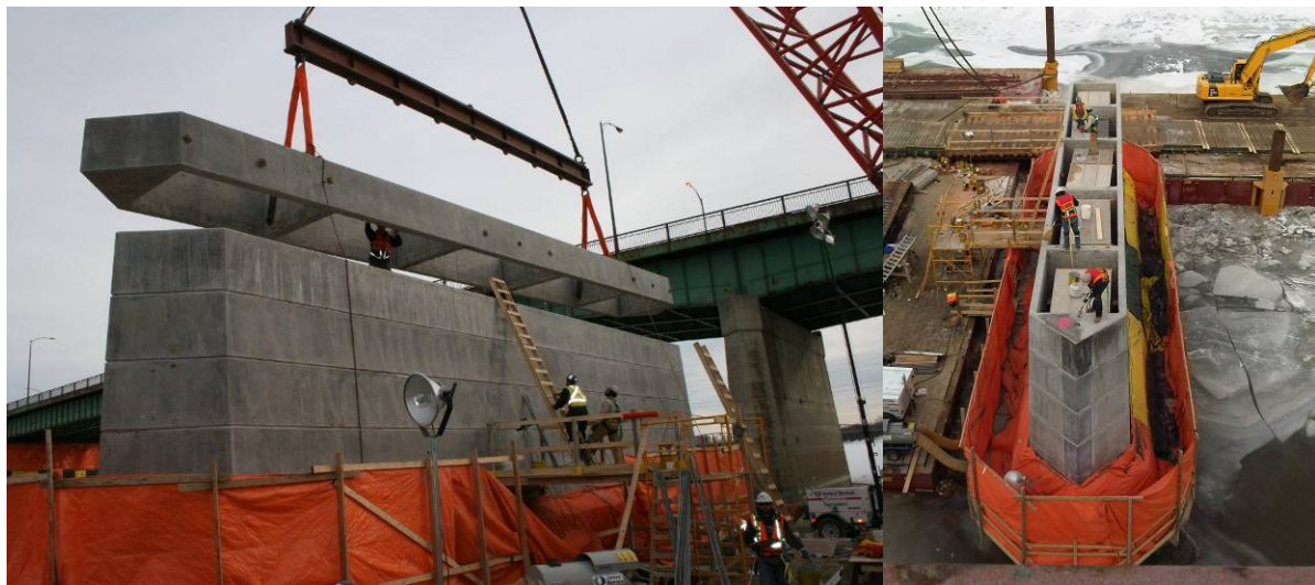
Figure 5 - Construction of River Piers
