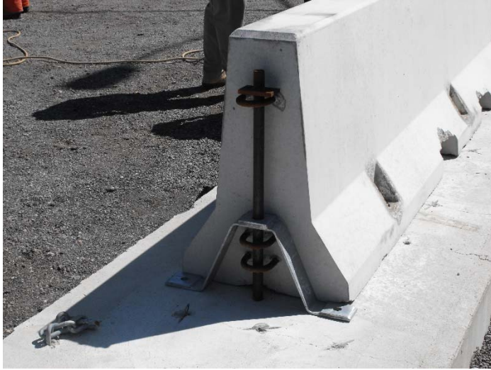
Figure 2: Type M Temporary Concrete Barrier Strapped to Concrete (MTO File Photo)
