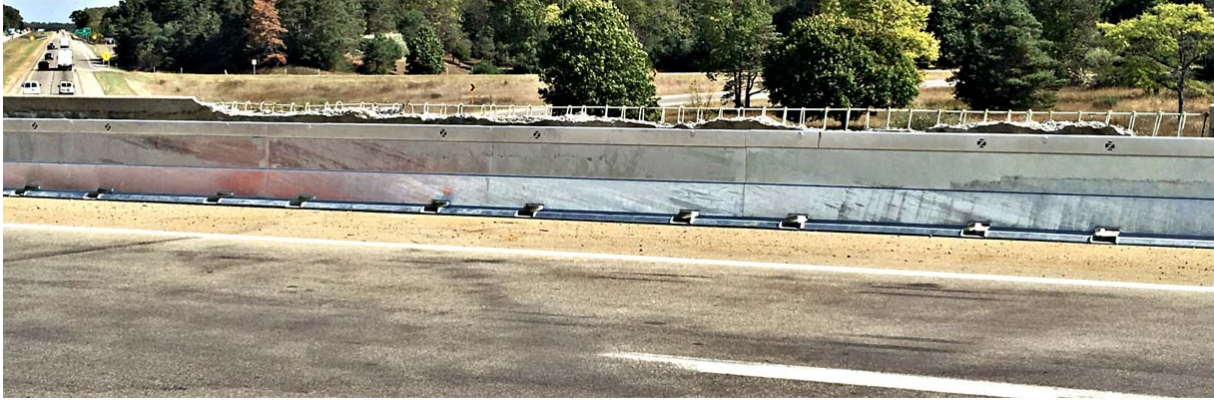
Figure 4: ZoneGuard Temporary Steel Barrier Installation [19]
