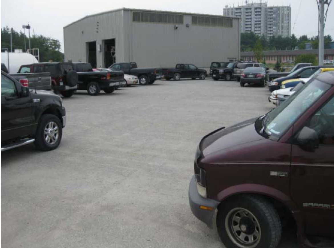
Figure 2. A pervious concrete parking lot in Georgetown, Ontario [2].
