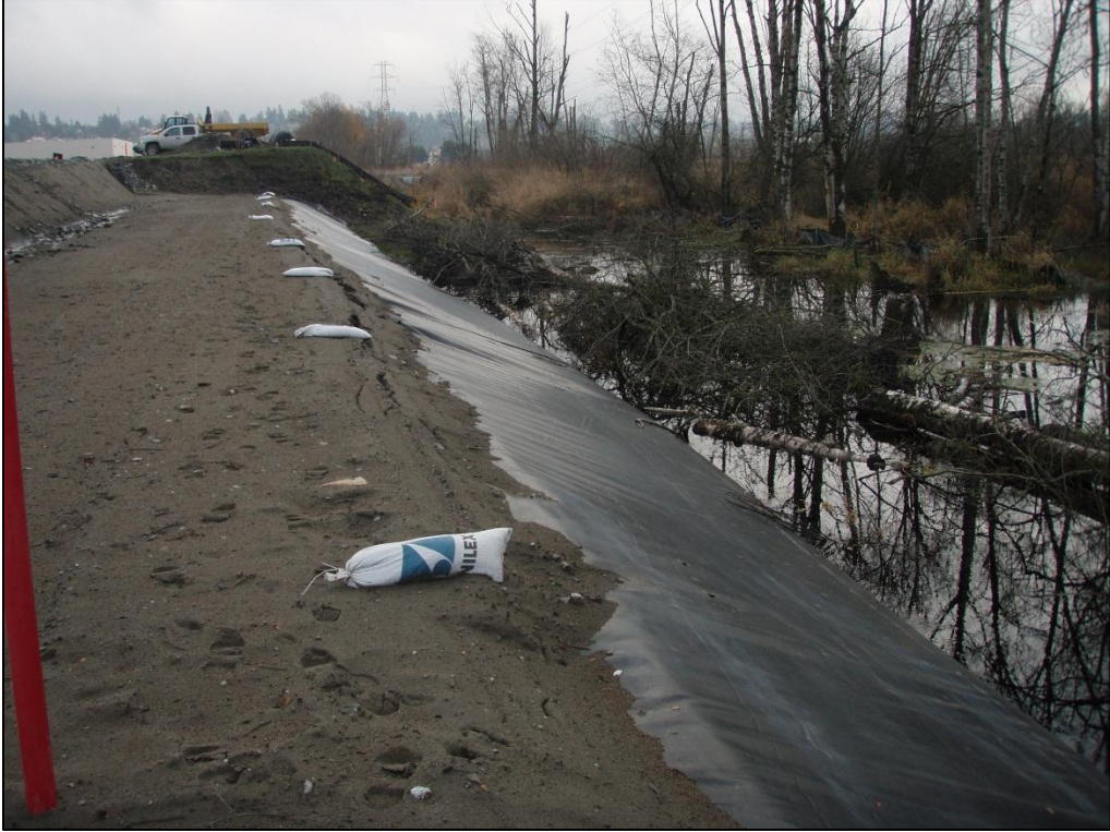
Photo 3. Separation berm along northern periphery of Burns Bog, under construction.
