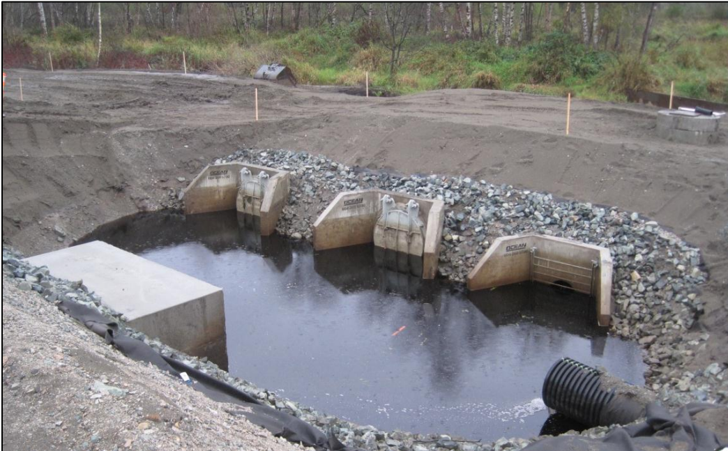
Photo 1. Water control structure installed facing south.
