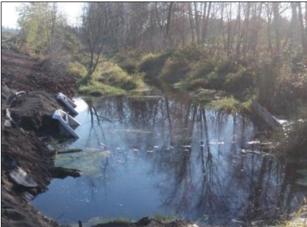
Photo 2. Water control structure installed, facing southeast.
