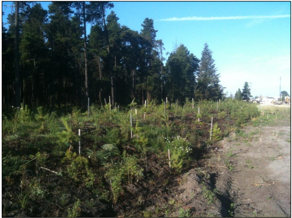
Photo 4. Separation berm along northern periphery of Burns Bog, completed and planted.
