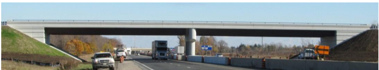
Fig. 10: Westminster Drive Underpass over Hwy 401 with integral abutments and integral pier
