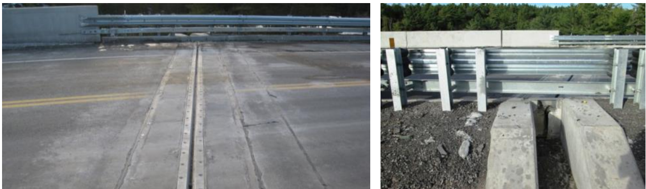
Fig. 21: Expansion joint at the end of an approach slab
