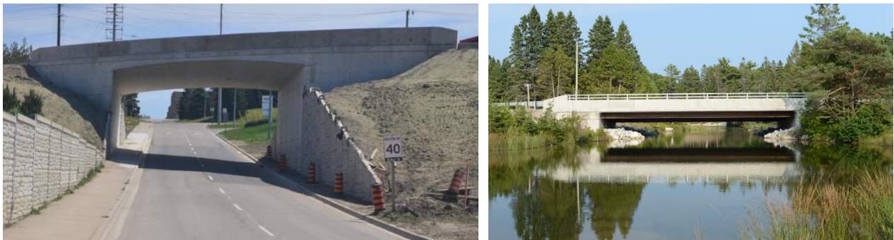
Fig. 1. Single span rigid frame bridge (left) and single span integral abutment bridge (right)
