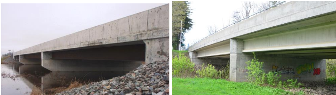
Fig. 9: Steel and precast concrete I-girder bridge with integral abutments and integral piers
