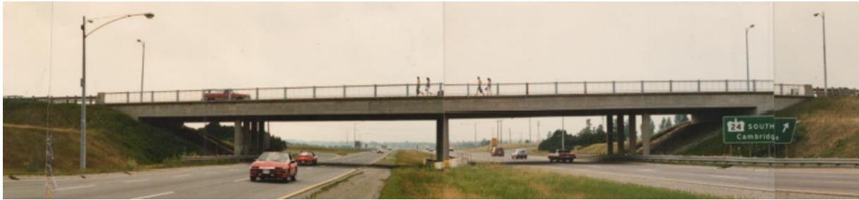
Fig. 2. Hespeler Rd Underpass over Hwy 401, an integral abutment bridge in Ontario built 1962
