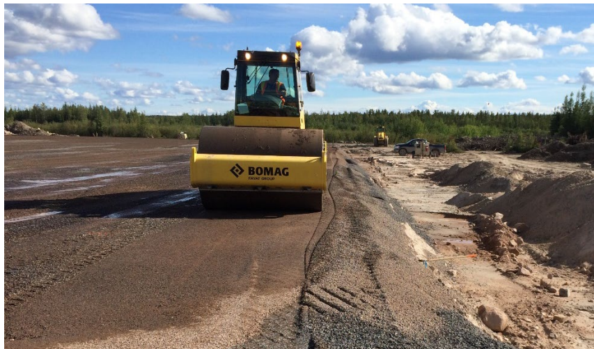
Figure 5 – Granular Base Course Construction Stony Rapids Airport 2014
