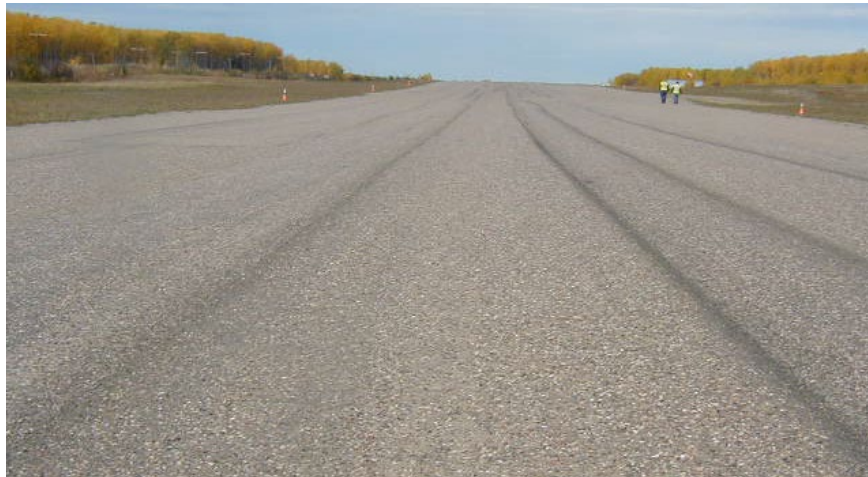
Figure 6 – Newly Completed Seal Coat on a Runway
