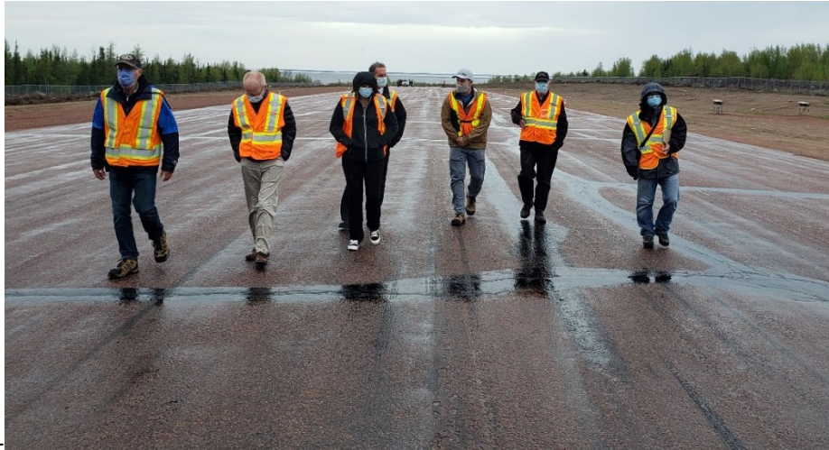
Figure 4 – Surface Inspection of Wollaston Lake Airport Runway June 2021
