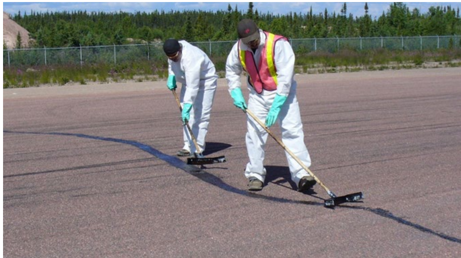
Figure 7 – Crack Sealing Using Rubberized Crack Sealant
