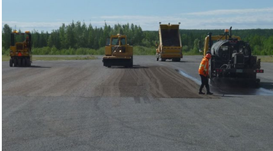
Figure 8 – Maintenance Crews Spot Sealing the Runway
