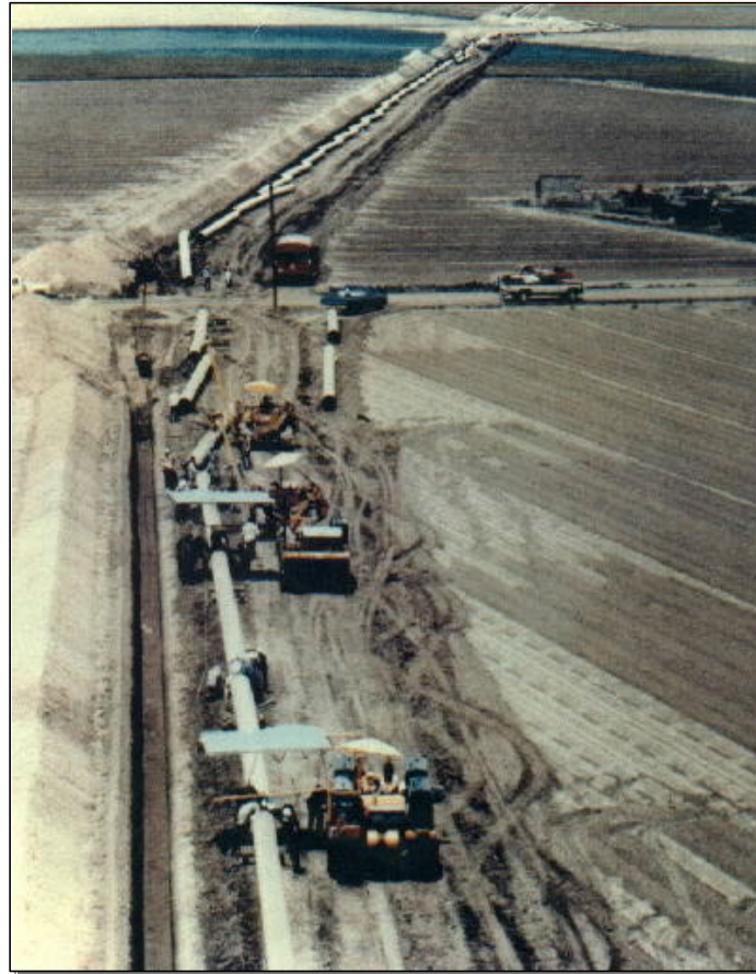
Figure 3.1 Pipeline Construction Spread Associated with Rural Environment Open Field Construction
