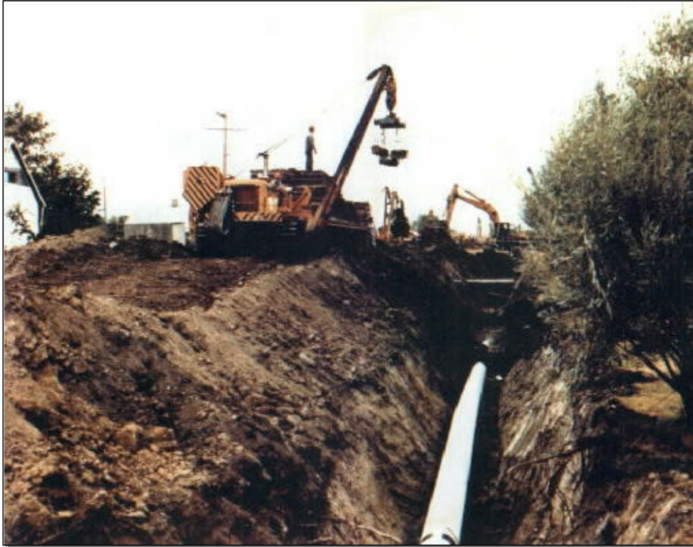
Figure 3.3 Pipeline Construction Spread – Working Off the Flattened Spoil Pile
