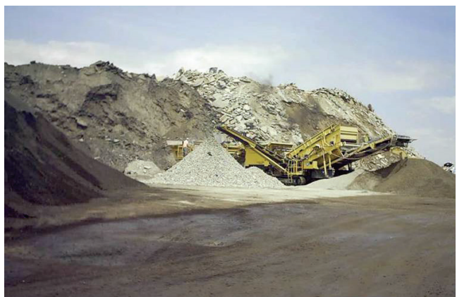
Photograph C14-2 Processing of Reclaimed Concrete Material
