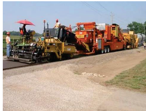
Photograph C13-3 - Paver-Laid surface recycling foamed asphalt train
