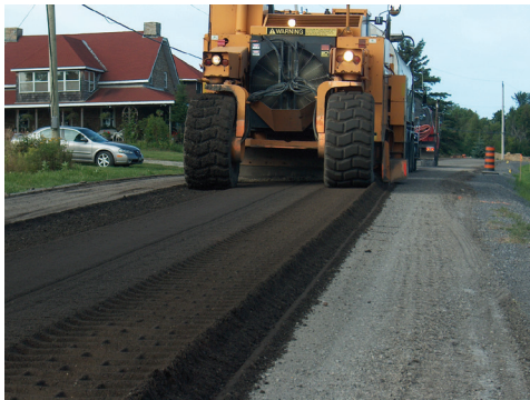
Photograph C13-2 - Conventional full-depth foamed asphalt stabilization unit
