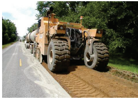
Photograph C13-5 - Full depth reclamation with cement stabilization
