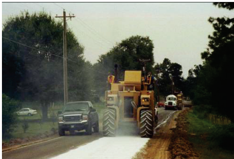
Photograph C13-4 - Full depth reclamation with lime stabilization
