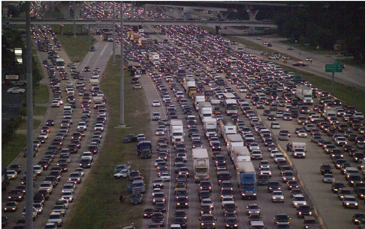
Figure 2: Reversible Flow Lane Operation during the Evacuation of Houston TX (Source: http://en.wikipedia.org/wiki/Image:RitaHoustonEvacuation.jpg – Accessed in November 2008)
