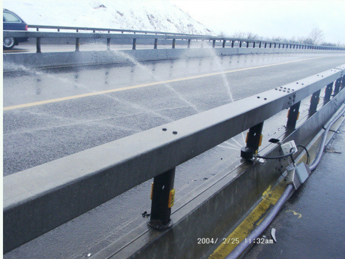
De-icing agents spraying system in a road work
