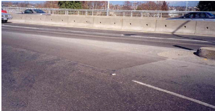
15. Asphalt Concrete Distress Area of Oak Street Bridge 1995 Deck Rehabilitation (Photograph 1) Sheet Membrane Waterproofing System, Vancouver, 1998.
