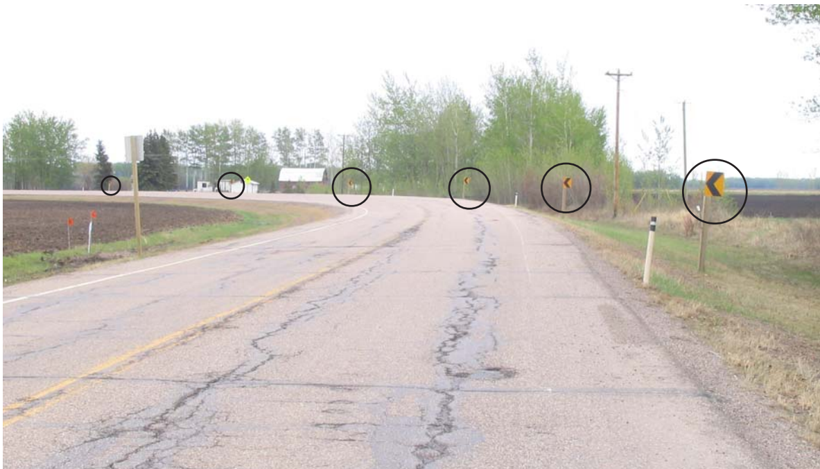
Photo taken on an unlit two-lane undivided rural roadway. Six chevron alignment signs are mounted on the outside of the curve. An access road to a development is located along the curve.
