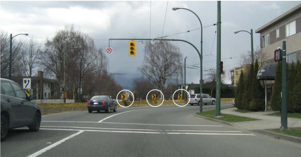
Photo taken on a multi-lane urban roadway along a divided section. Three Chevron Alignment signs are mounted on the centre median.
