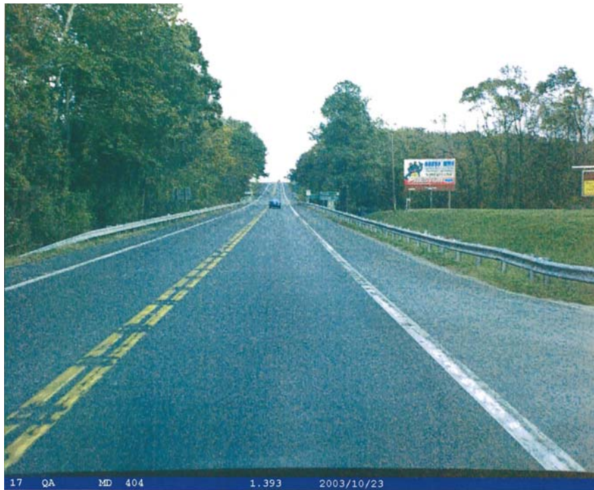
Figure 8: CLRS implemented in a Maryland no passing zone (Photo courtesy: Thomas Hicks)
