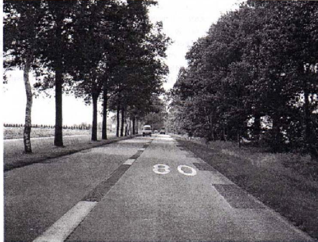
Figure 10: Raised Centreline Rumble Strips in the Netherlands (8)
