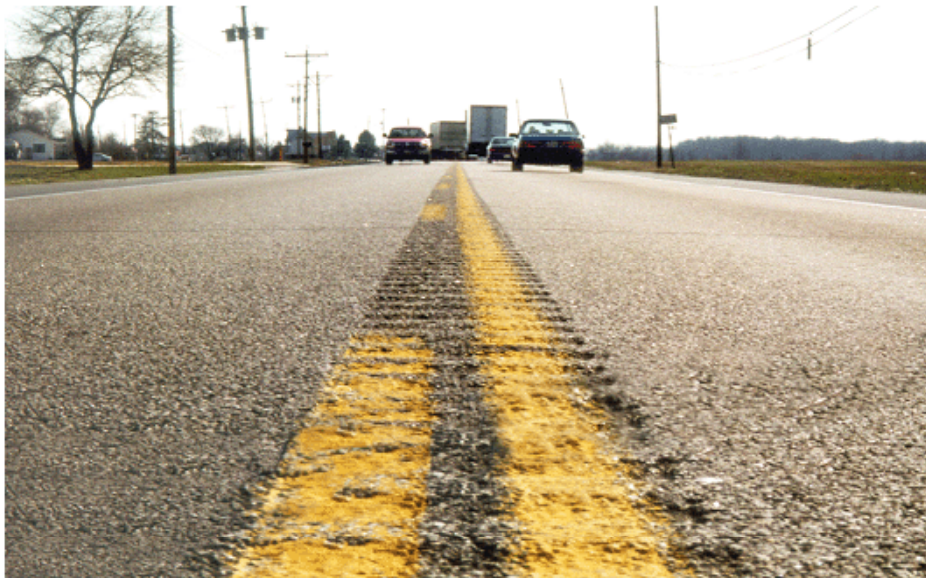
Figure 6: Delaware CLRS installation in passing zone (13) ( http://www.deldot.net/static/projects/rumblestrip/index.html )
