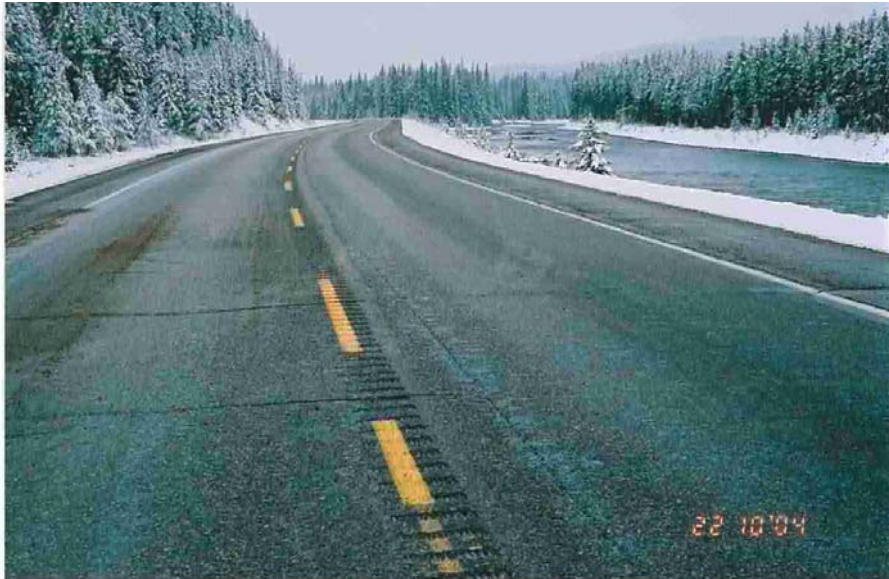
Figure 4: CLRS installed on the TransCanada Highway regardless of passing zone (Photo: Dr. John Morrall)
