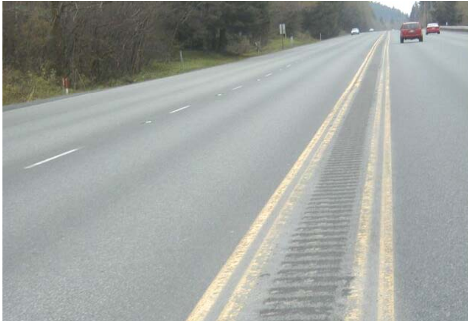
Figure 11: Oregon CLRS installed in a flush median on Mt. Hood Highway (2)
